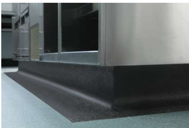
Figure 2: Example of a plinth with coving
