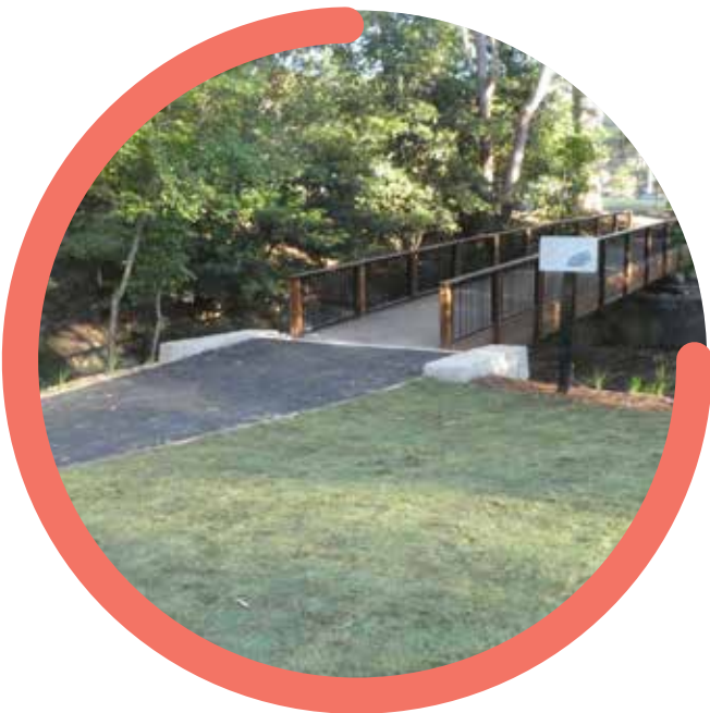
The timber pedestrian bridge at Bicentennial Park, West Pymble was replaced with a wider version to improve accessibility.
