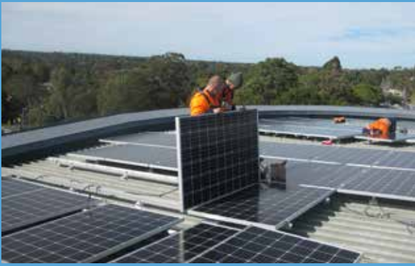
Solar PV panels being installed
