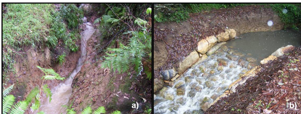
Figure 6: Upper tributary of Coups Creek at The Glade, Wahroonga a) illustrates incision through deep clay soil and b) construction of a rock ramp to control bed erosion.
