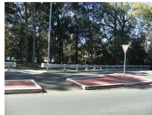
Stencil pavement on traffic medians.
