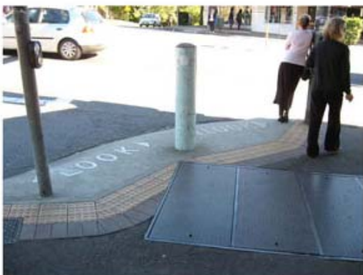
Ramp design requires ugly bollard not aligned with service lids.
