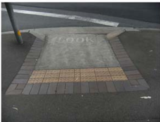
Concrete ramp with tactile pavers in asphalt pavement with brick trim.
