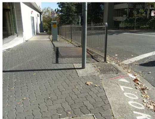
Interlocking pavers designed for vehicle use exist on footpaths.
