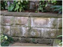
*Figure 8 Cracks resulting from minor movement.*
