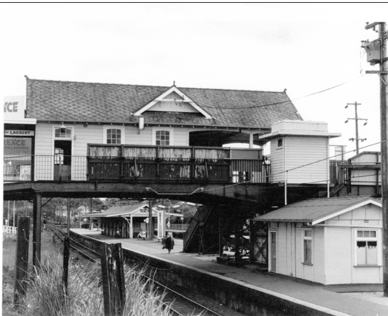
Lindfield Station showing original overhead booking office, 'haunched beams' and the very rare pre-cast signal box
