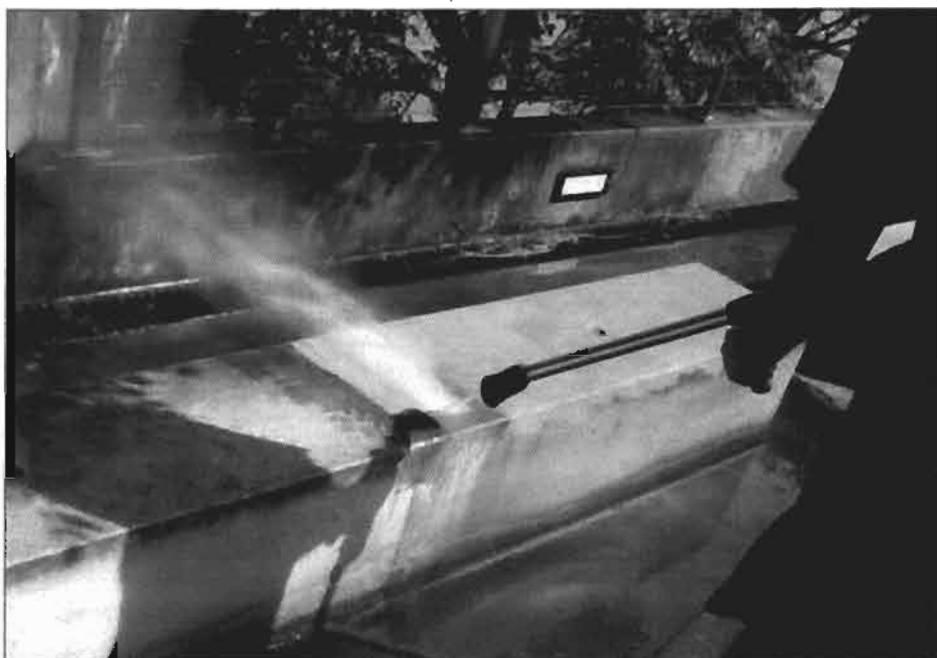
Cleaning and preparing the sandstone.
