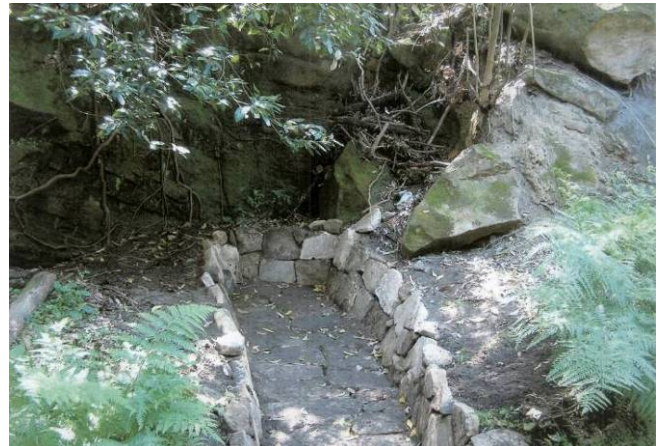
Left: The scoured stormwater channel prior to the ditch construction; Right: the improved stormwater ditch lined with stone pavers. Photos provided by Robert Dash.
