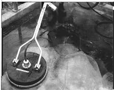
Cleaning and preparing the sandstone.
