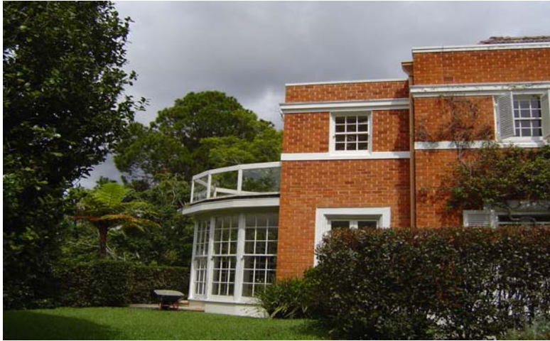
Fig. 7 Front façade of house looking at southern end with conservatory at ground floor and later balcony above. Upper floor over living room doors in centre of picture appears to be a later addition
