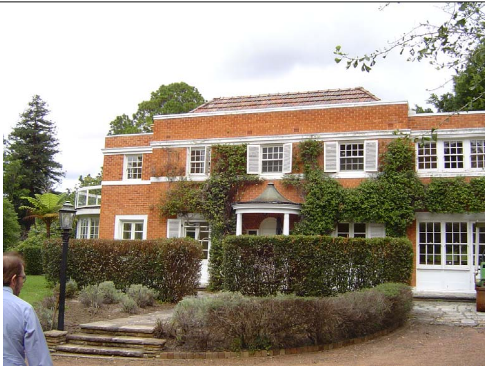
Fig.3 Front façade of house with centre symmetrical section containing upper bedrooms and ground floor entrance as original first floor section of house. The single window to the left and triple windows to the right appear as a later addition to first floor. Note high brick parapet with hipped tile roof behind.
