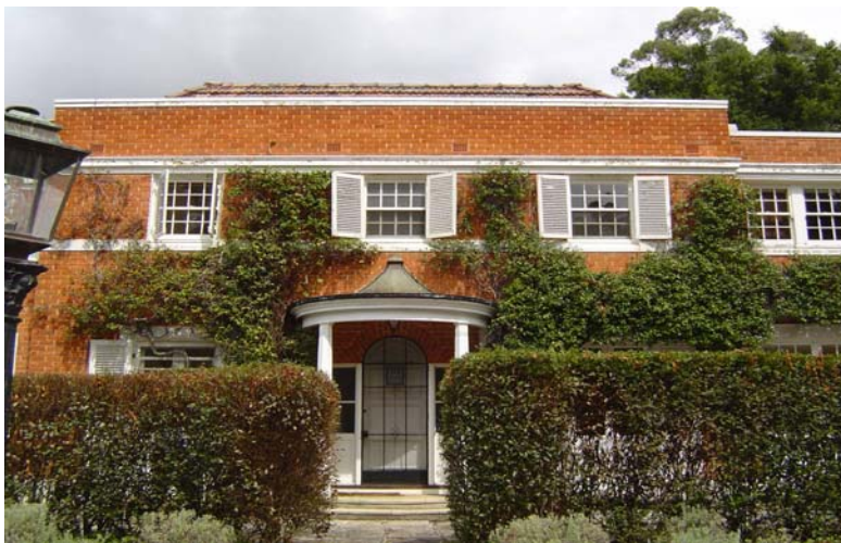
Fig. 3 Front façade of 49-51 Billyard Avenue. Note terra cotta tile hip roof just visible behind parapet. Front entrance with curved copper roofed porch and columns.
