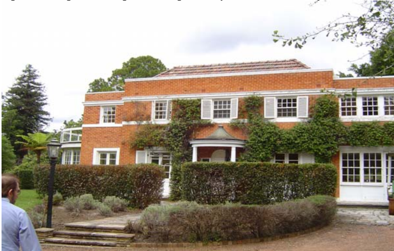
Fig. 6 Front façade of red brick house showing terraced garden in front of residence Note: Large ground floor windows to right side possibly replaced original garage door opening.
