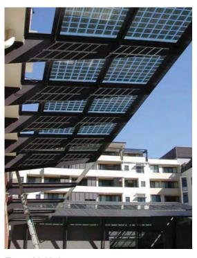
Figure 3A.18-4: Photovoltaic cells integrated into the awning design.
