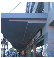
Figure 3A.11-4: Suspended steel box section type awning with under awning lighting.
