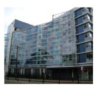
Figure 3A.20-2: Glazed facade to minimise sound infiltration into the building.
