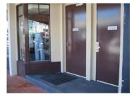
Figure 3A.9-1: Fire doors integrated as part of the shopfront design with matching colour scheme.
