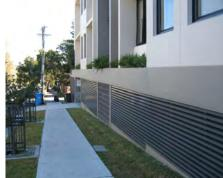
Figure 4.9-2: Ventilation grilles to basement car park are well integrated with overall facade design.
