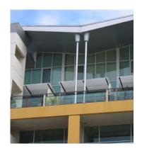
Figure 3A.6-3: Drainage pipes integrated with the overall facade design.
