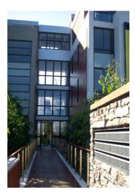
Figure 3C.22-2: Extensive use of glazing to stairway area to provide natural light.
