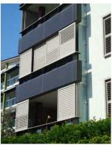
Figure 4.5-3: Louvres and sliding panels as an integrated facade element.
