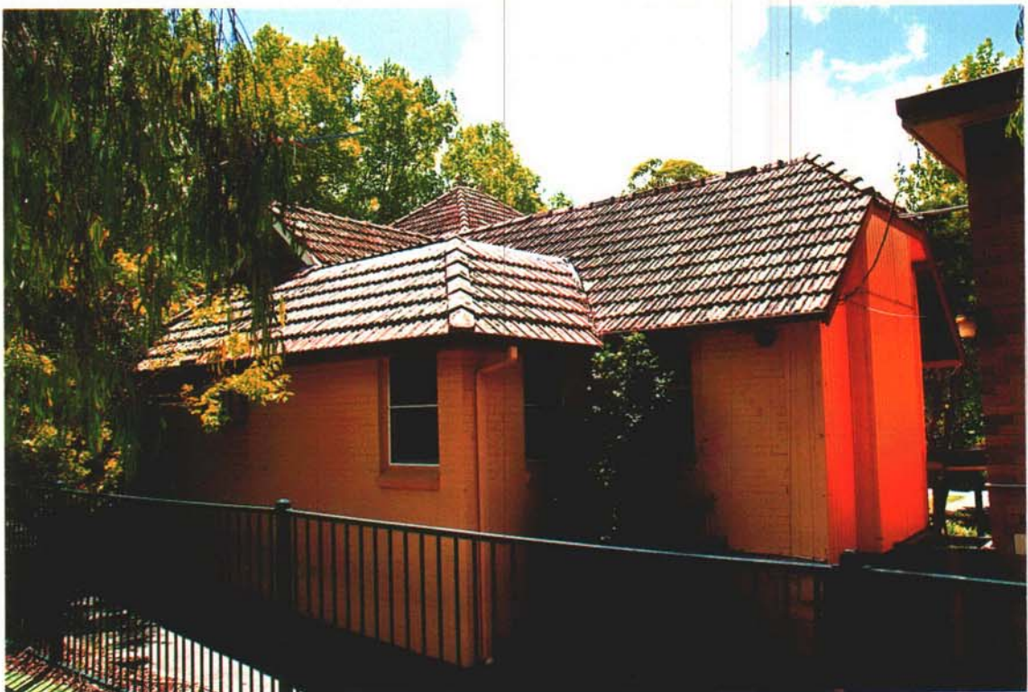
Figs. 8&9 –Unsympathetic addition to west elevation running awkwardly across original projecting bay & gable
