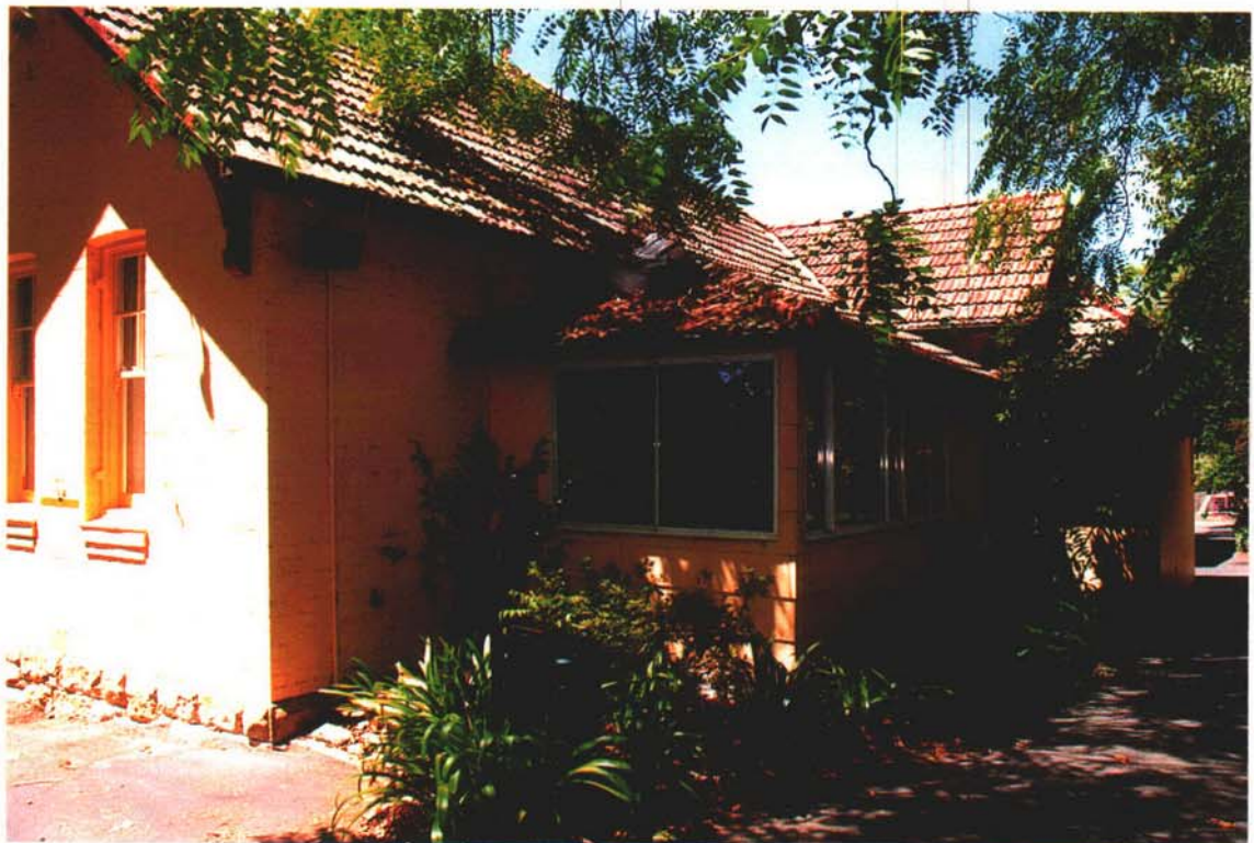
Fig. 7 – Sub standard addition on west side near north east corner replacing original verandah
