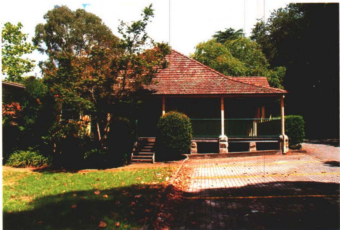
Figs. 4&5 – Front elevation) and east side elevation showing stone base, pier bases, timber columns and simple timber hand railing & side steps
