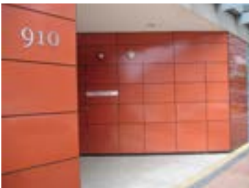
Figure 12.1-1: Building identification sign
