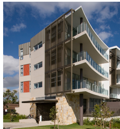
Figure 7C6-6: Distinct form to highlight the building corner.
