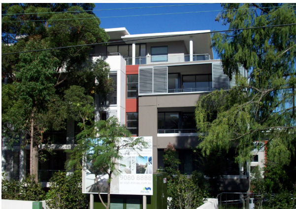
Figure 7C.6-3: Well articulated building facade with the use of balconies. Sun shading devices incorporated into the balcony design for solar access control.
