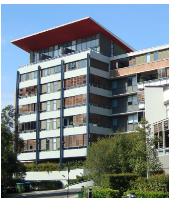
Figure 7C.8-4: Distinctive roof design.
