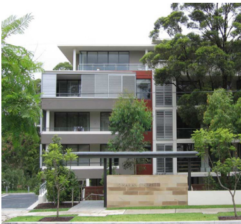
Figure 7C.8-3: The upper storeys of the building articulated with mezzanine penthouse.
