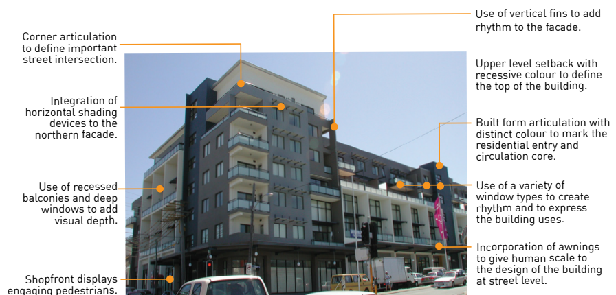
Figure 8C.9-2: Methods of achieving building articulation and modulation.
