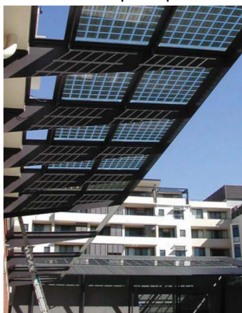
Figure 8C.9-3: Photovoltaic cells integrated into the awning design.
