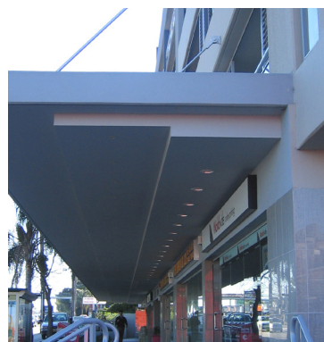
Figure 8C.11-3: Suspended steel box section awning with under awning lighting.
