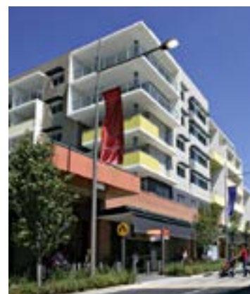
Figure 23.9-2: Use of a mix of solid and transparent balustrades on different levels to ensure visual privacy.
