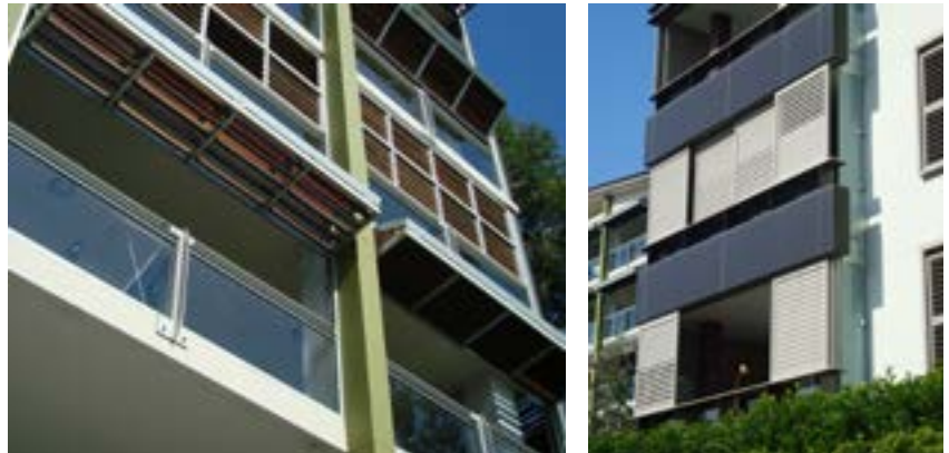
Figure 23.4-3: Louvres and sliding panels as an integrated facade element.
