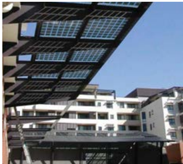
Figure 23.2-1: Photovoltaic cells integrated into the awning design.
