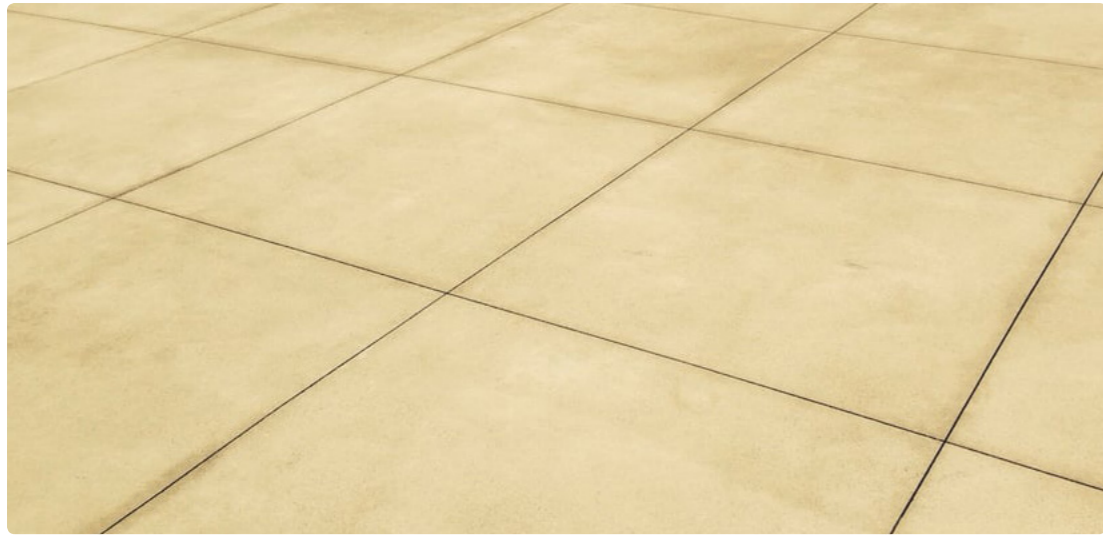
Coloured concrete with decorative sawcuts to main paths
