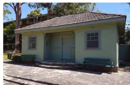
Figure 06 - Existing Tennis Pavilion
