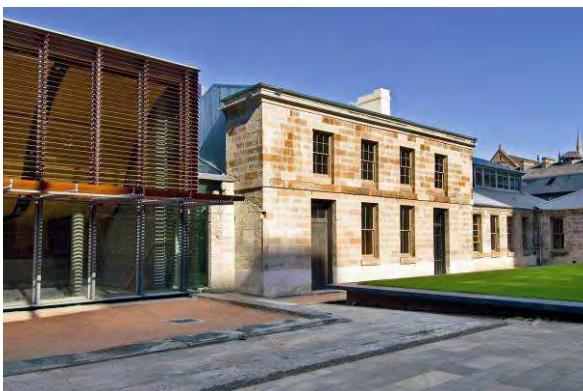
From top: Walsh Bay Wharves, c.1921, once a major shipping port, now a vibrant apartment, theatre and restaurant precinct; Burberry, Sydney, converted from major bank headquarters, c.1925; Burberry interiors re-using bank tellers, seats and desks; The Mint, Sydney, c.1855, where colonial coins were made, now offices.
