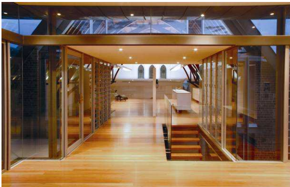
Above: Demonstrating these tips in practice for a church conversion into two homes: Toxteth Church, Glebe. The new internal structure inserted into the old church for new mezzanine levels was built in a way that allows its future removal without damaging heritage fabric (tip 8). The old roof structure is used as a feature in the new design (tip 3). A rear modern pavilion addition is discrete and lightweight (tip 4). Open courtyards separate the church and hall from the new addition, allowing the old building to remain prominent (tip 6).
