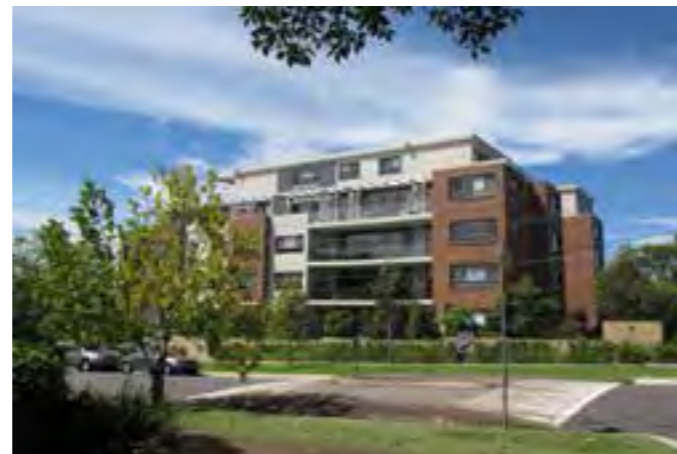
(R) Tyron Road Apartment Development
