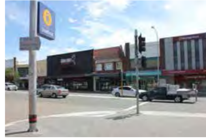
19 Retail development adjacent to Pacific Highway movement corridor
