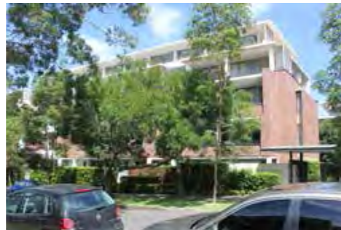
14 5 storey height Tyron Road residential development
