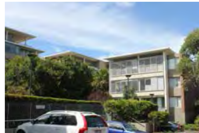
(R) Tyron Road Apartment Development
