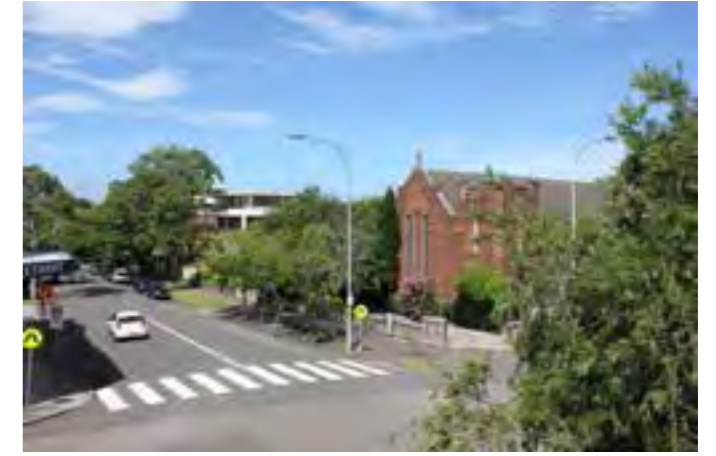
20 Street condition of Lindfield Avenue and Tyron Road
