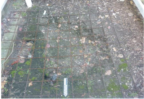
Figure 3.4 Surface of the well site is covered with a protective wire mesh. (Source: GML 2015)
