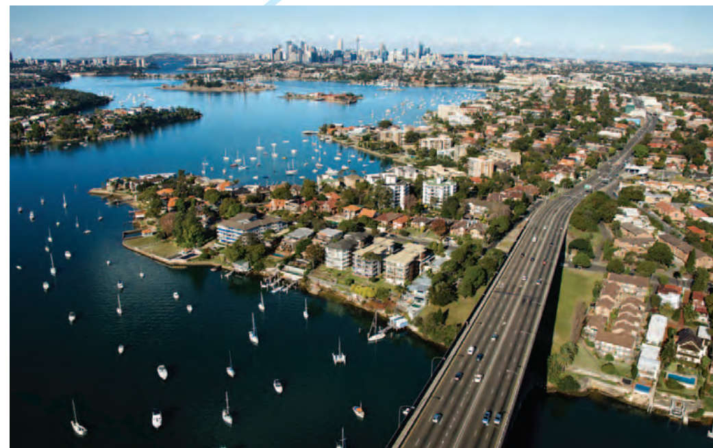
Gladesville Bridge, Victoria Rd, Drummoyne
