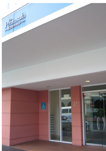
Figure 12.2-1: Street name and number displayed prominently near the building entry
