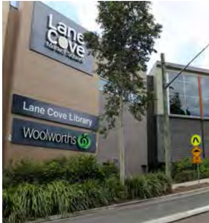
03 Austin Street frontage
