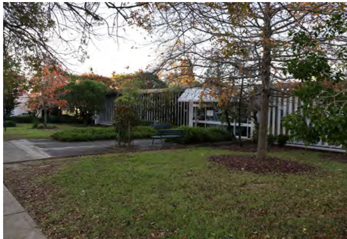
Figure 23. 01 View of the Library from the Pacific Highway
