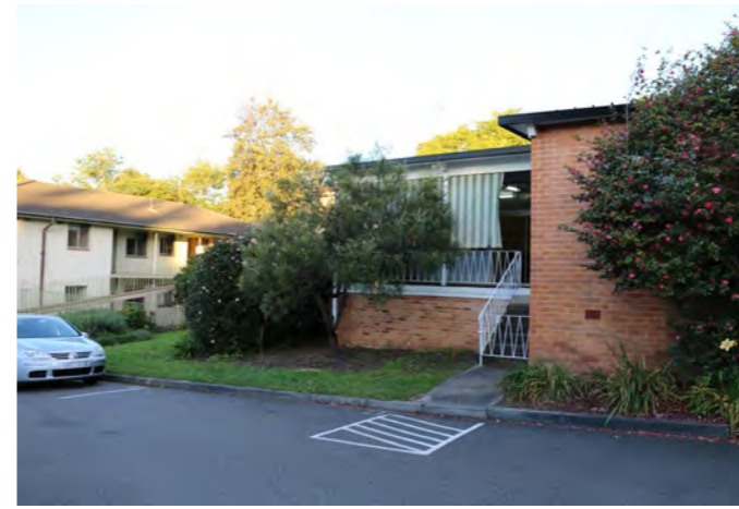
Figure 16. 03 View of the Ku-ring-gai Centre for Community
