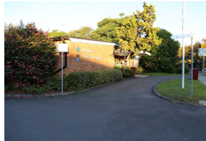
Figure 15. 02 View of the Ku-ring-gai Centre for Community
