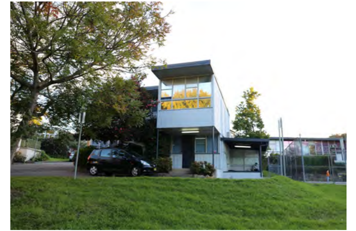
Figure 20. 08 View looking west towards the rear of the library & KYOS
