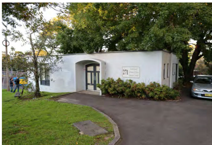
Figure 25. 09 View of the Community Centre looking east
