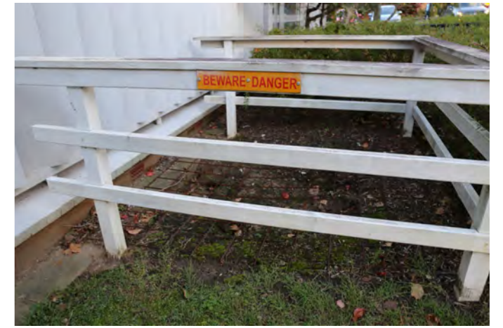
Figure 17. 04 View of the well located outside the library
