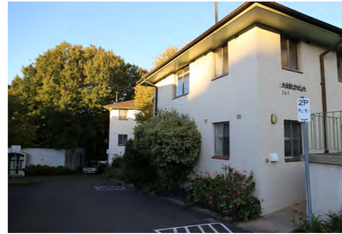
Figure 19. 07 View looking east towards the Community Centre and self-contained units
