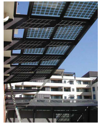
Figure 8C.1-3: Photovoltaic cells integrated into the awning design.
