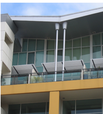
Figure 8C.9-4: Drainage pipes integrated with the overall facade design.
