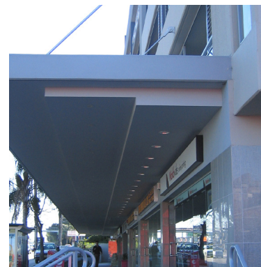
Figure 8C.11-3: Suspended steel box section awning with under awning lighting.
