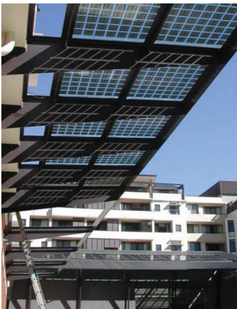
Figure 8C.9-3: Photovoltaic cells integrated into the awning design.
