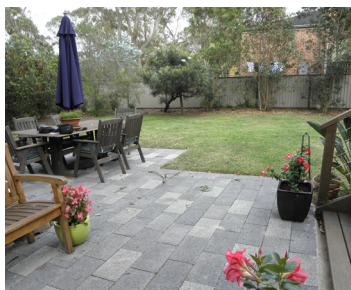
Figure 4B.3 -3 Permeable paving used to reduce runoff to bushland on a Location C property.
