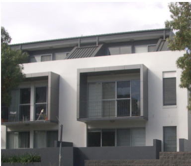
Figure 6C.10-1: Top floor setback with recessive colour scheme to minimise the bulk and scale.
