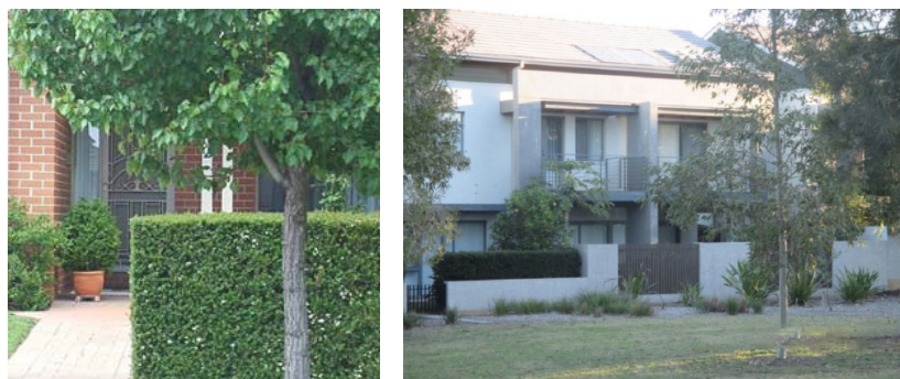
Figure 6C.15-2: Use of hedges as fencing.
