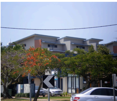
Figure 6C.10-2 Broken roof forms on townhouses
