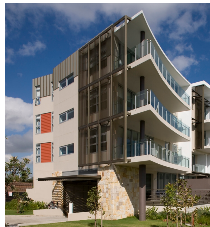
Figure 7C.6-6: Distinct form to highlight the building corner.
