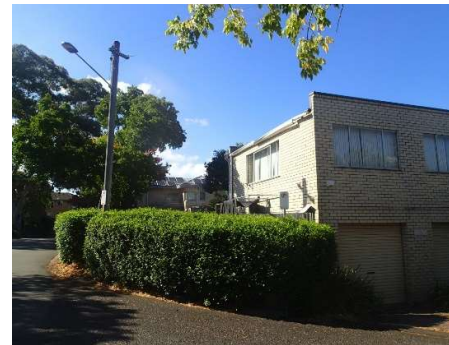
Figure 19 - The rear and east side elevations of the two-storey garage structure of Killiecrankie viewed from Larkin Lane.
