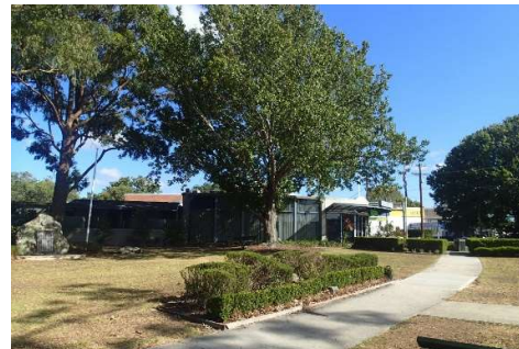
Figure 13 - View north from the Roseville Memorial Park to the subjects site.
