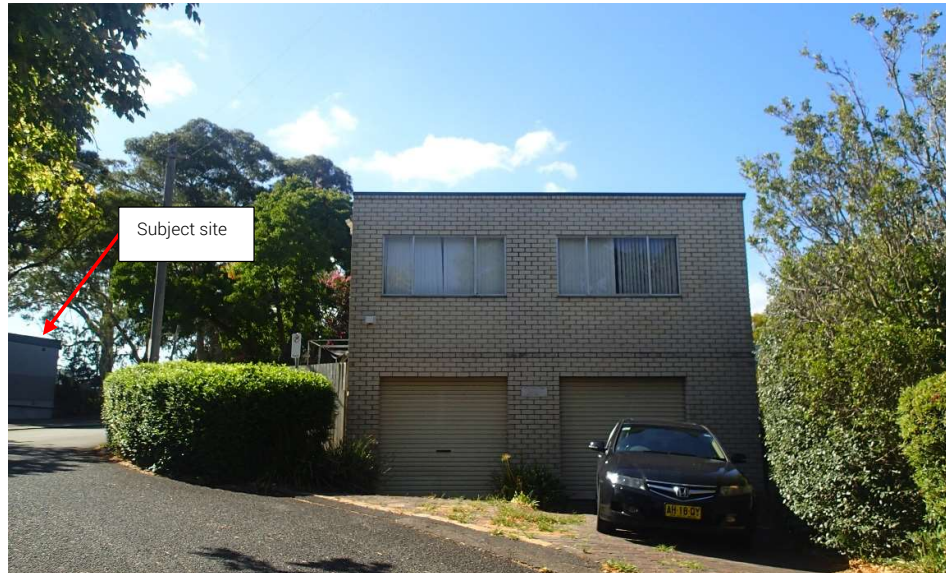
Figure 20 - Rear elevation of the two-storey garage structure viewed from Larkin Lane with the subject site seen in the distance, identified by the red arrow.
