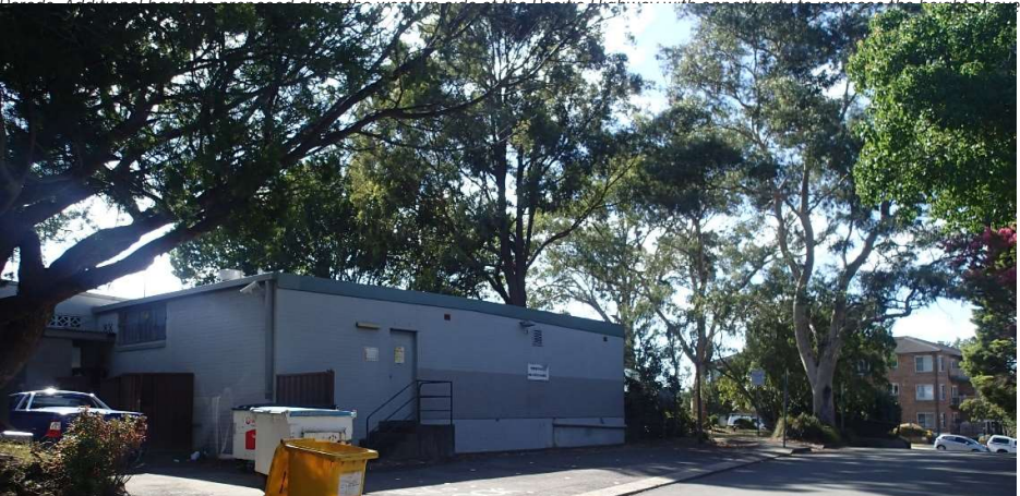
Figure 11 - The rear western frontage of the subject site addressing Larkin Lane.
