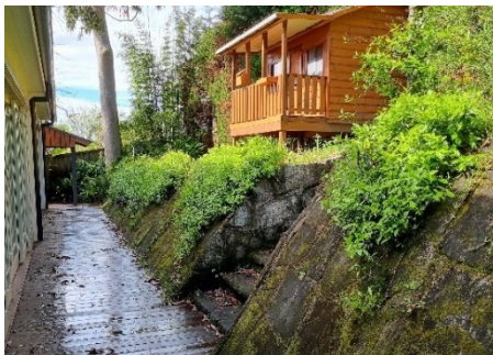
28 Original stone bank to rear and steps.
