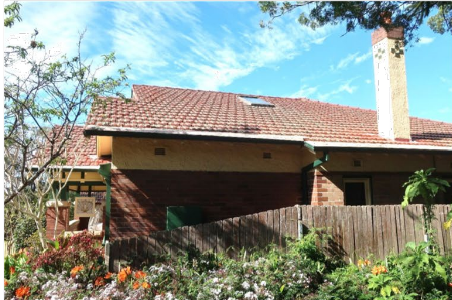
Figure 3-4 The northern side of the house facing Khartoum Lane. Note the non-original skylight
