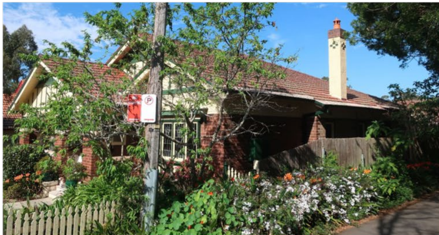
Figure 3-1 The house at 10 Rosedale Road, with Khartoum Lane on the right (northern side)
