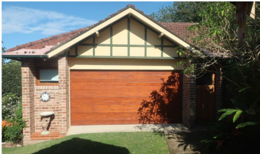
Figure 3-2 The garage, looking west
