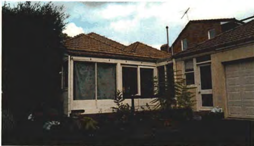
Figure 12 View of the rear of the house showing the verandah infill and the garage which appears to have been a mid twentieth century building converted c1980s. Source Paul Davies Pty Ltd July 2009.
