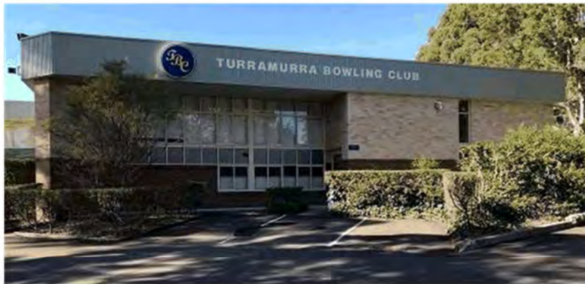
Turramurra Bowling Club Building (Source: https://www.vennu.com.au )
