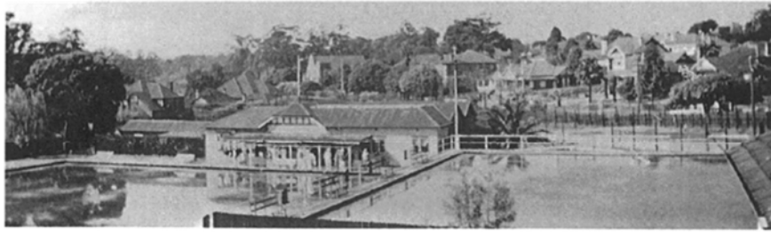
The Bowling greens flooded in April 1942. A storm-water drain on the southern side of No 2 green collapsed after a storm leaving an opening 6 ft wide and 50 ft long. Photo: courtesy of the Killara Bowling Club
