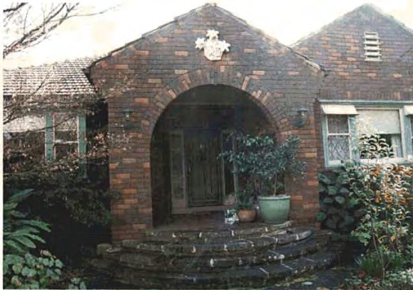
Figure 14 View of the front porch where the bay was removed to install stone steps. Source Paul Davies Pty Ltd July 2009.
