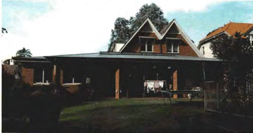
Figure 21 View of the rear of No 16 showing the substantial rear addition and changes to the roof form to create the attic rooms. Source Paul Davies Pty Ltd July 2009.
