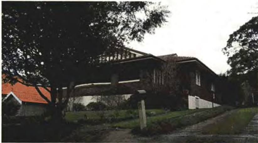
Figure 28 A large and impressive interwar house at 25 Wandella St which has no heritage protection. Source Paul Davies Pty Ltd July 2009.
