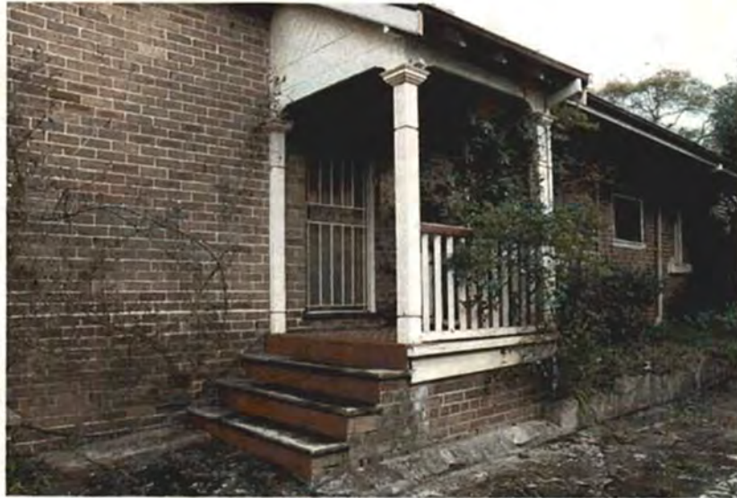
Figure 10 Figure 11 View of the interior of the side porch. The details appear to be contemporary to the construction of the house except for the poorly fitted treads and risers. Source Paul Davies Pty Ltd July 2009.
