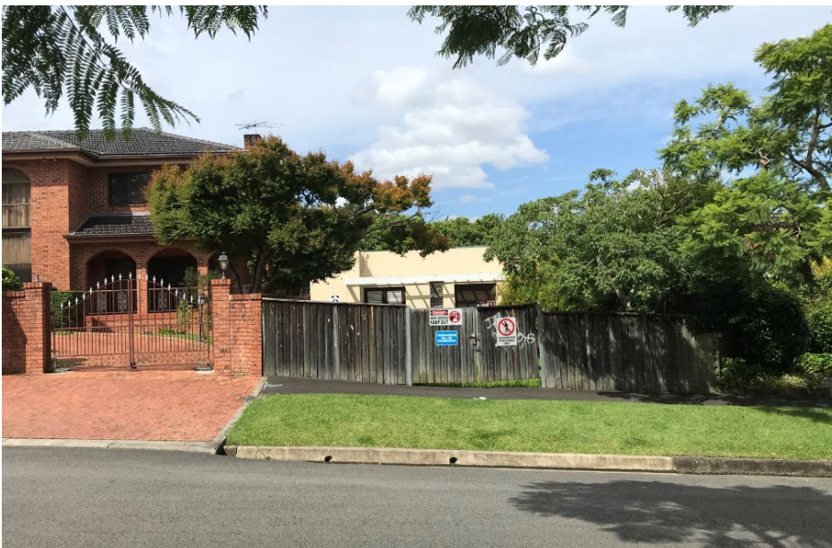
Above: Substation No. 590 streetscape view
