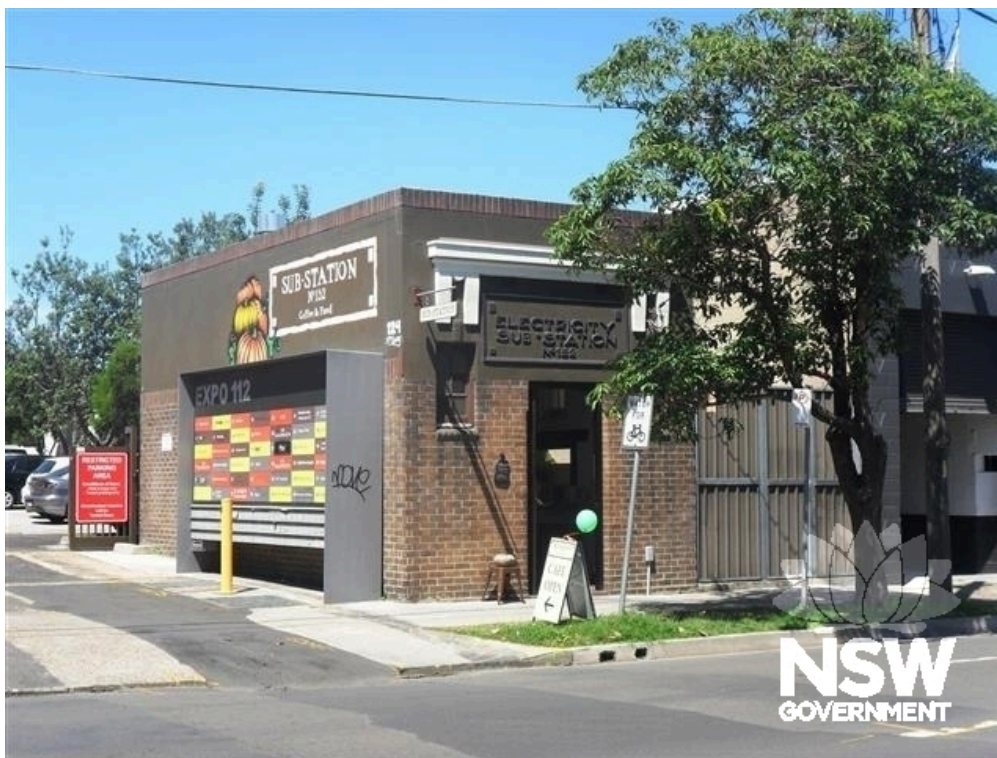
Above: Example of a substation cafe conversion in Alexandria (source: State Heritage Inventory)
