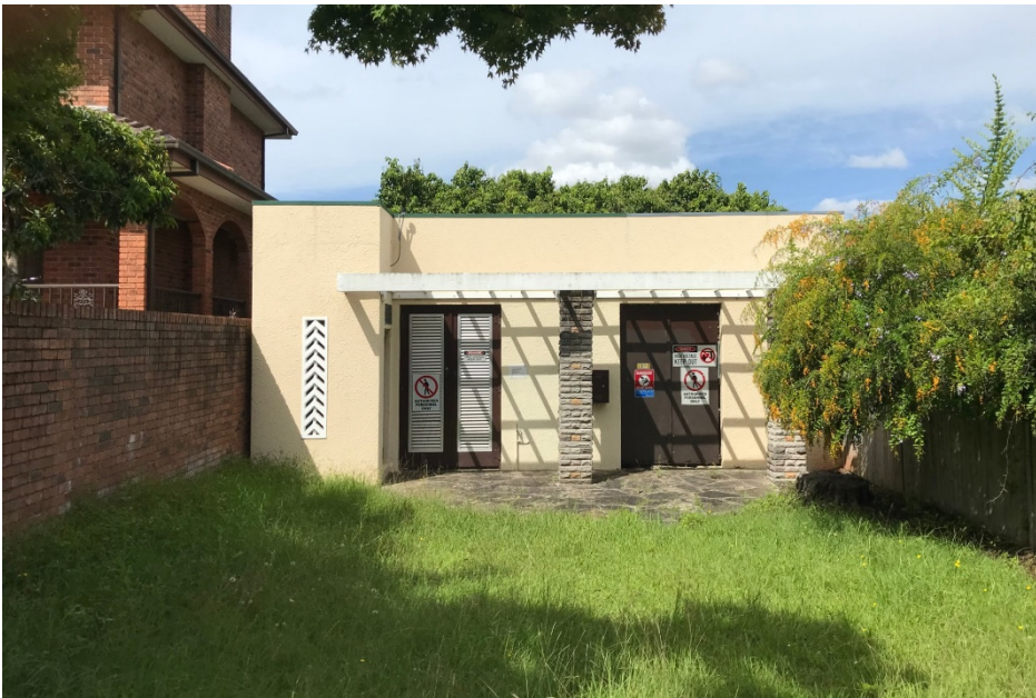
Above: Substation No. 590 streetscape front elevation
