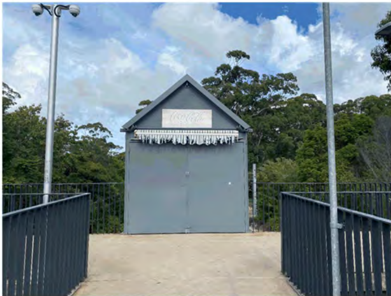
Figure 1-4 Cantilevered retail kiosk (currently not leased) located on the footbridge
