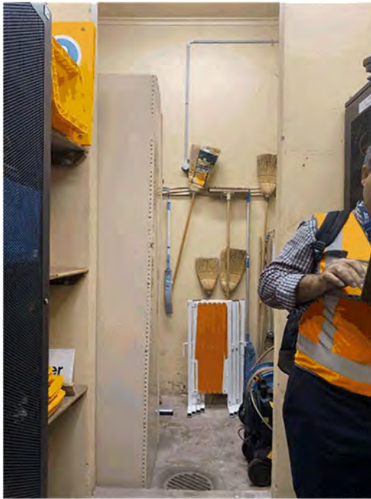
Figure 4-16 Internal layout of communications/store room, Killara Station, looking north (AECOM, 2021)
