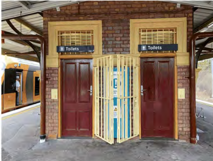
Figure 4-14 Northern end of station building modified to include toilets (AECOM, 2021)
