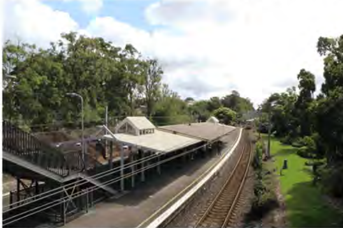
Figure 4-11 Killara Station looking south, with "up" line (Platform 1) in foreground (AECOM, 2021)
