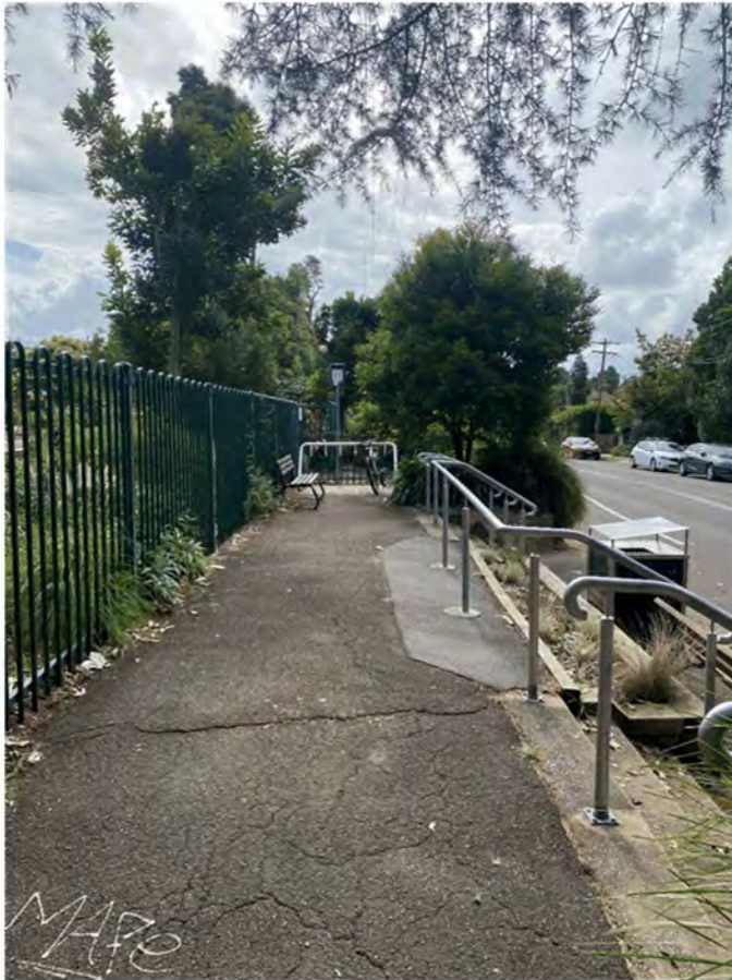
Figure 1-10 Werona Avenue footpath and bus stop seating area
