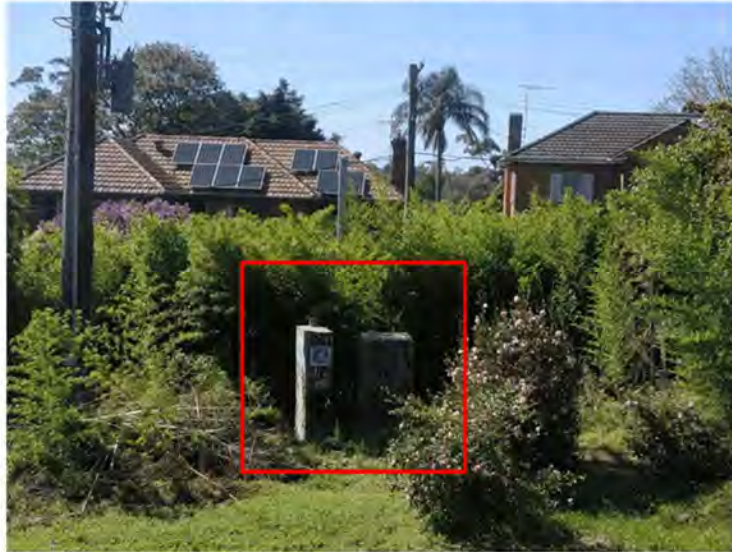
Figure 6-12 Vegetation to be trimmed or removed around the existing transformer
