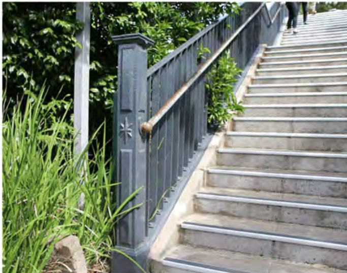
Figure 4-5 Original star patterned newel posts, balustrades and handrails at the Werona Avenue (eastern) access to footbridge. These are also present on the Culworth Avenue side of the footbridge (AECOM, 2021)
