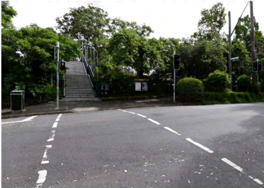
Figure 4-1 Existing entrance to Killara Station from Werona Avenue (AECOM, 2021)
