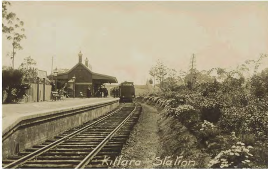
Figure 3-4 Killara Railway Station prior to duplication, looking south. Note piling fence at left (State Library of Victoria)
