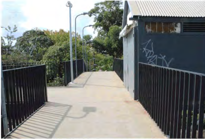
Figure 4-8 Deck of footbridge, looking east. Cantilevered kiosk is at right (AECOM, 2021)
