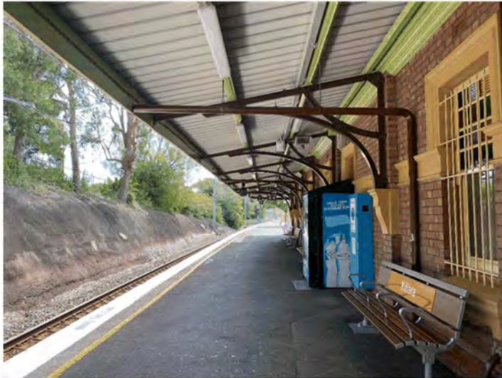
Figure 4-12 Station building on "down" line (Platform 2), looking north (AECOM, 2021)
