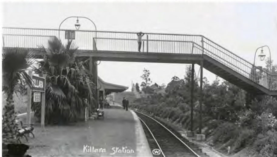
Figure 3-5 Killara Railway Station following duplication and construction of footbridge, c.1910 (National Library of Australia)
