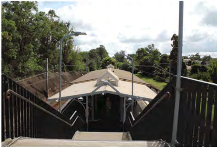
Figure 4-13 Modified roofline of main station building and contemporary canopy addition in foreground, looking north from footbridge (AECOM, 2021)
