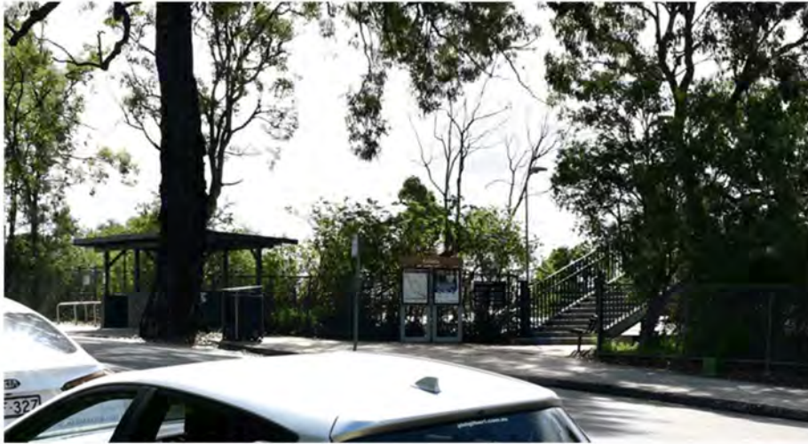
Figure 4-2 Existing entrance to Killara Station from Culworth Avenue (AECOM, 2021)
