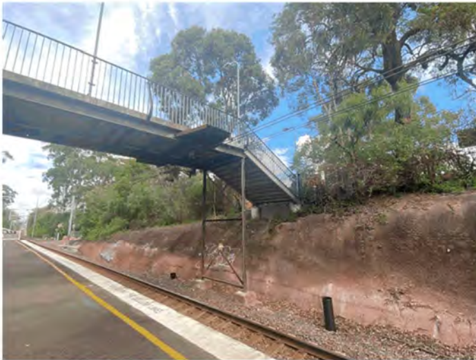
Figure 4-9 Footbridge, looking south toward Culworth Avenue from platform (AECOM, 2021)
