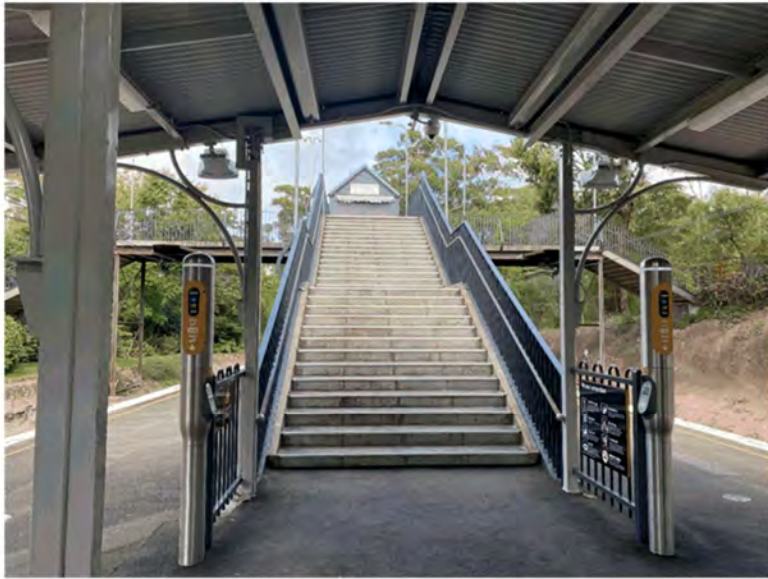
Figure 1-3 Platform stairs and footbridge
