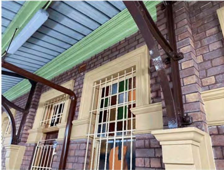
Figure 4-18 Windows in station building (AECOM, 2021)
