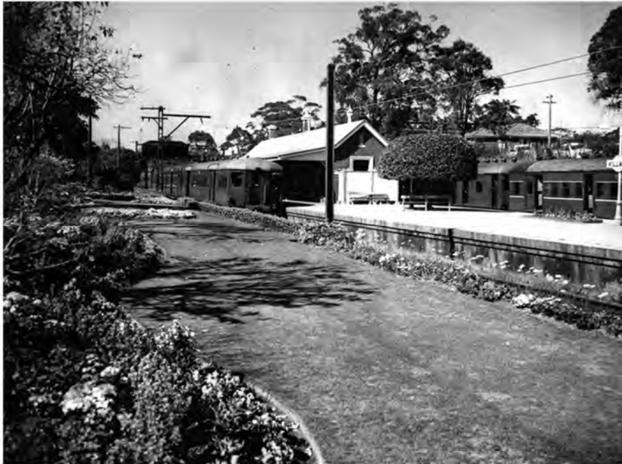
Figure 6-14 Killara Station looking south, undated (Australian Railway Historical Society NSW, Image 008774)
