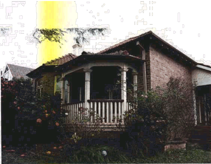
Figure 8 View of the front of No 10 showing the front verandah and the side porch. Source Paul Davies Pty Ltd July 2009.
