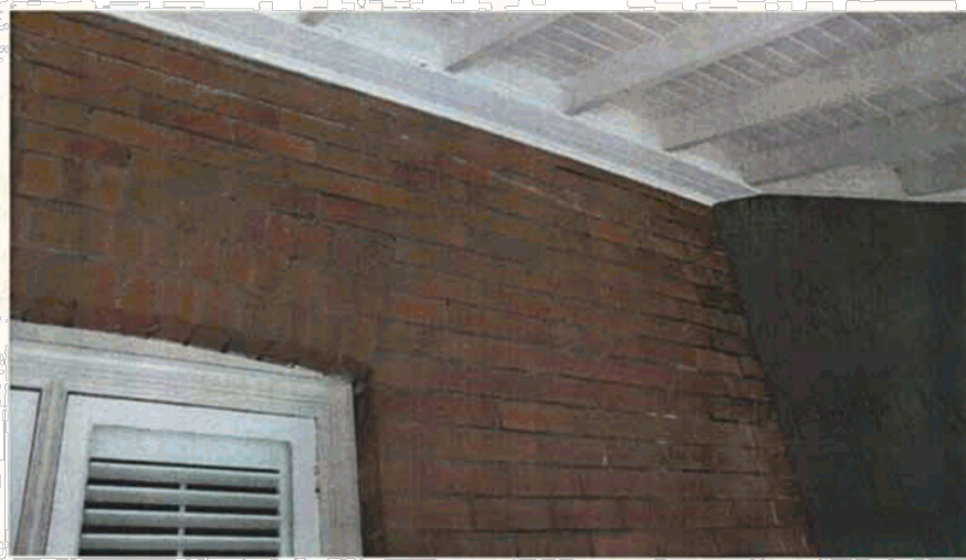
Figure 20 View within the front verandah of No 16 showing the silhouette of the original verandah post and beam. Source Paul Davies Pty Ltd July 2009.
