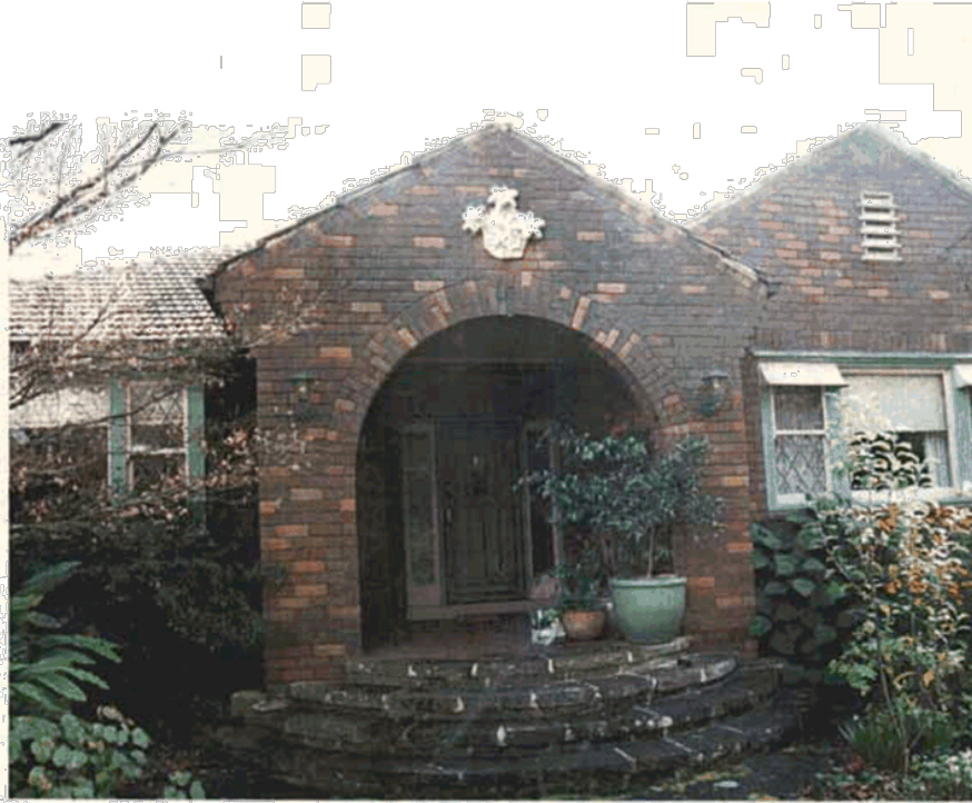
Figure 14 View of the front porch where the bay was removed to install stone steps. Source Paul Davies Pty Ltd July 2009.
