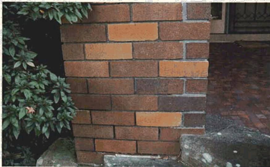
Figure 15 Detailed view of the front porch showing the stitch marks in darker mortar and bricks where the bay was removed to install the stone steps. Source Paul Davies Pty Ltd July 2009.
