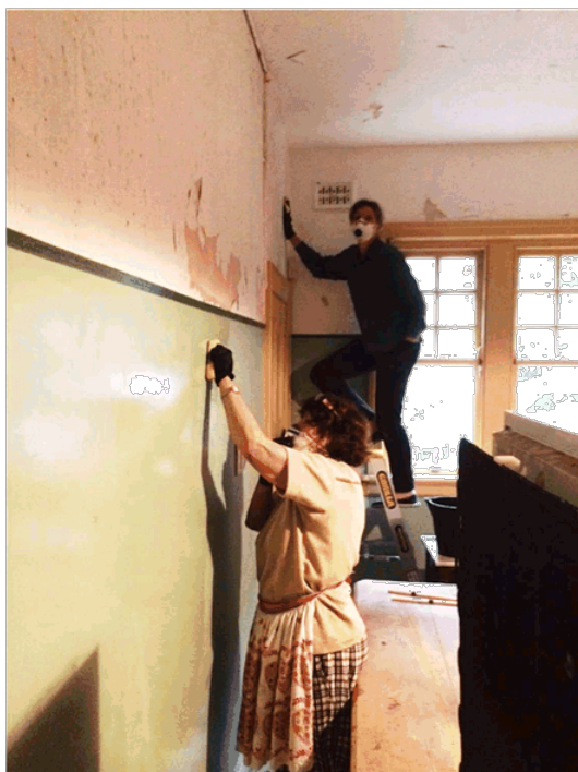
Volunteers removing mould in kitchen
