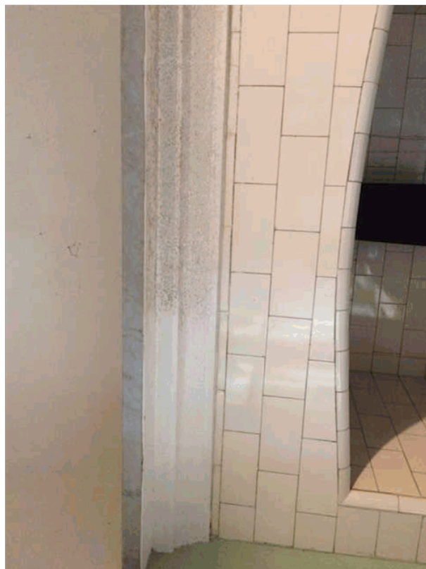
Mould damage
