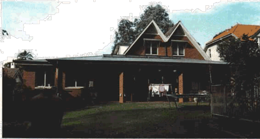
Figure 21 View of the rear of No 16 showing the substantial rear addition and changes to the roof form to create the attic rooms. Source Paul Davies Pty Ltd July 2009.
