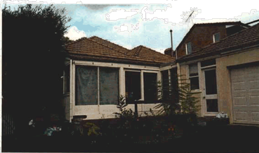
Figure 12 View of the rear of the house showing the verandah infill and the garage which appears to have been a mid twentieth century building converted c1980s. Source Paul Davies Pty Ltd July 2009.
