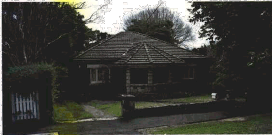
Figure 26 No. 10 Bancroft Ave which has been proposed an individual heritage item but which is now included in the draft conservation area 14. The property appears as an intact representative example of an interwar residence. Source Paul Davies Pty Ltd July 2009.
