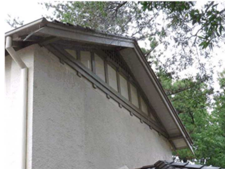
Figure 3.21 The eastern gable of the chapel wing. The shadow in the stucco below shows the location of the window that was originally located in this wall. (Source: GML 2017)
