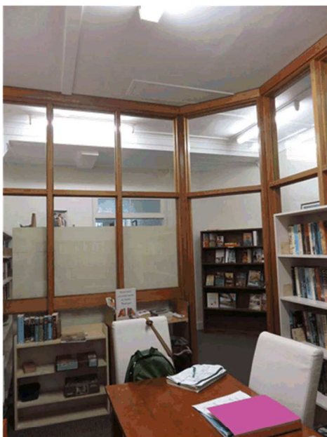
Figure 3.30 The contemporary glazed screen wall that divides the room. (Source: GML 2017)
