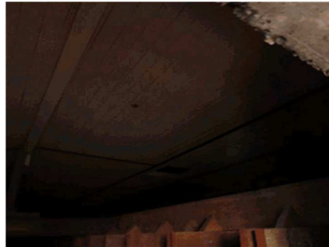
Figure 3.46 The original boarded ceiling remains above the newer cedar ceiling in the chapel. The dark lines possibly indicate the former location of walls. (Source: GML 2017)
