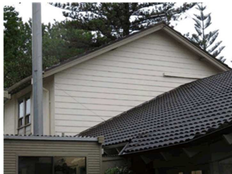
Figure 3.16 The boarded gable is the only part of the south elevation of the main part of the building that is visible. The brown tiled roof in the foreground is part of the 1980s building. (Source: GML 2017)
