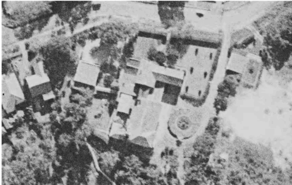
Figure 2.27 1956 aerial of the subject site showing buildings and immediate gardens, including established gardens on the tennis court, grotto and garage, of the Lourdes Hospital. (Source: LPI NSW)
