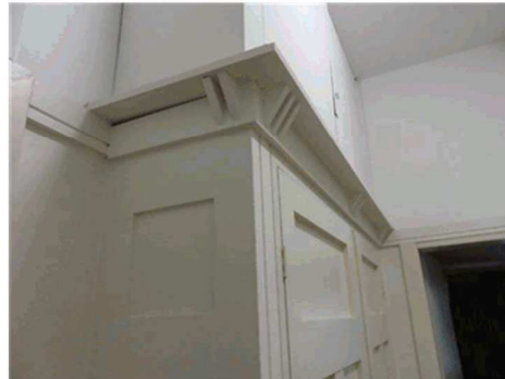
Figure 3.35 The joinery unit in the upper landing, which appears to have been relocated from elsewhere in the building. (Source: GML 2017)
