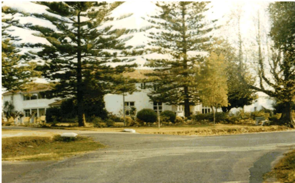
Figure 2.24 The site c1960s, published in Cook, KM 1991, The Railway Came to Ku-ring-gai , Genlin Investments, Pymble. (Source: Ku-ring-gai Historical Society photographic collection)
