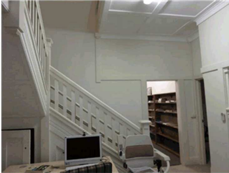
Figure 3.22 The entry lobby, looking towards the southern wall. (Source: GML 2017)
