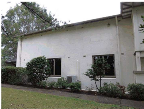
Figure 3.18 The north (front) elevation of the chapel wing. 'Shadows' of former window openings can be seen in the stucco finish. (Source: GML 2017)
