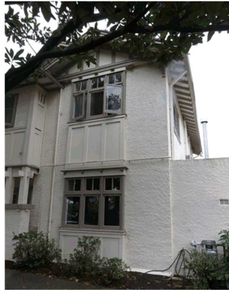
Figure 3.9 The framed wall panels below the windows on the north (front) elevation of Headfort House. (Source: GML 2017)
