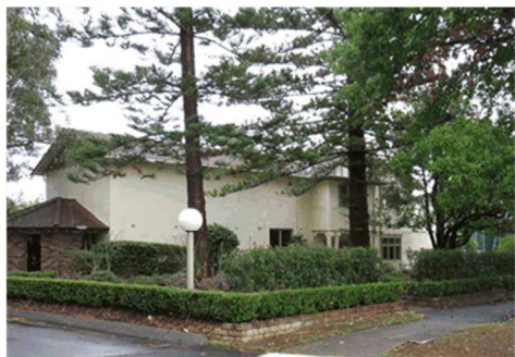
Figure 3.2 View of Headfort House from the northeast. The hedges around its front garden and large trees within the garden can be seen. (Source: GML 2017)
