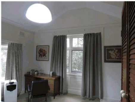
Figure 3.36 The wall of the bedroom. (Source: GML 2017)
