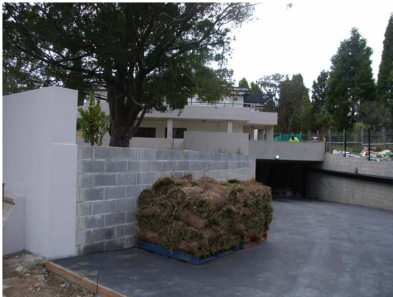
Photograph 2: View of driveway retaining walls from western (front) boundary
