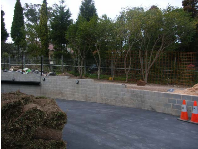
Photograph 3: View of driveway retaining wall and southern (side) boundary
