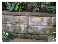
*Figure 8 Cracks resulting from minor movement.*
