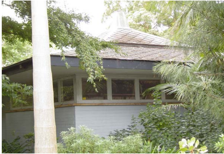
Fig 7 2 WirraClose Contemporary external photograph 2005. showing pyramidal roof and chimney of central pavilion Note original strip windows and wide eaves
