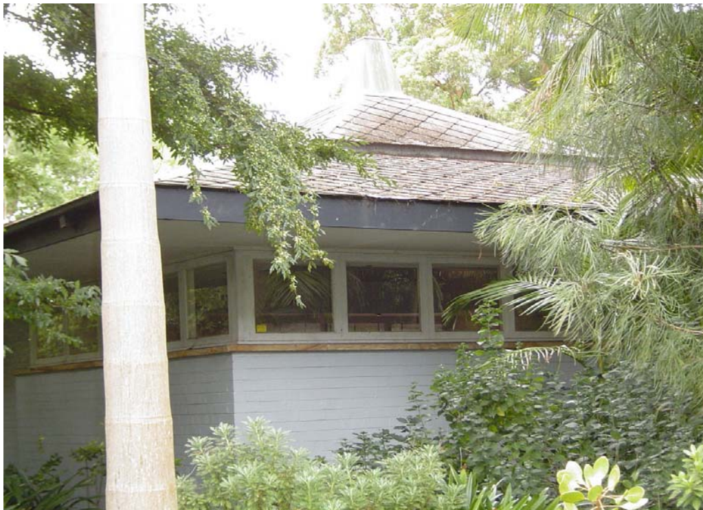
2 Wirra Close, St. Ives corner of house showing ventilation roof and central chimney, asbestos tiles, strip windows, wide eaves and sandstone sills May 2005
