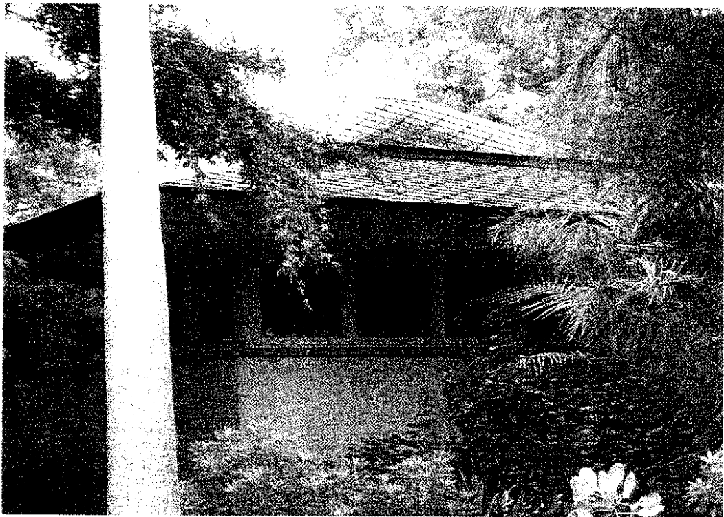
2 Wirra Close, St. Ives corner of house showing ventilation roof and central chimney, asbestos tiles, strip windows, wide eaves and sandstone sills May 2005
