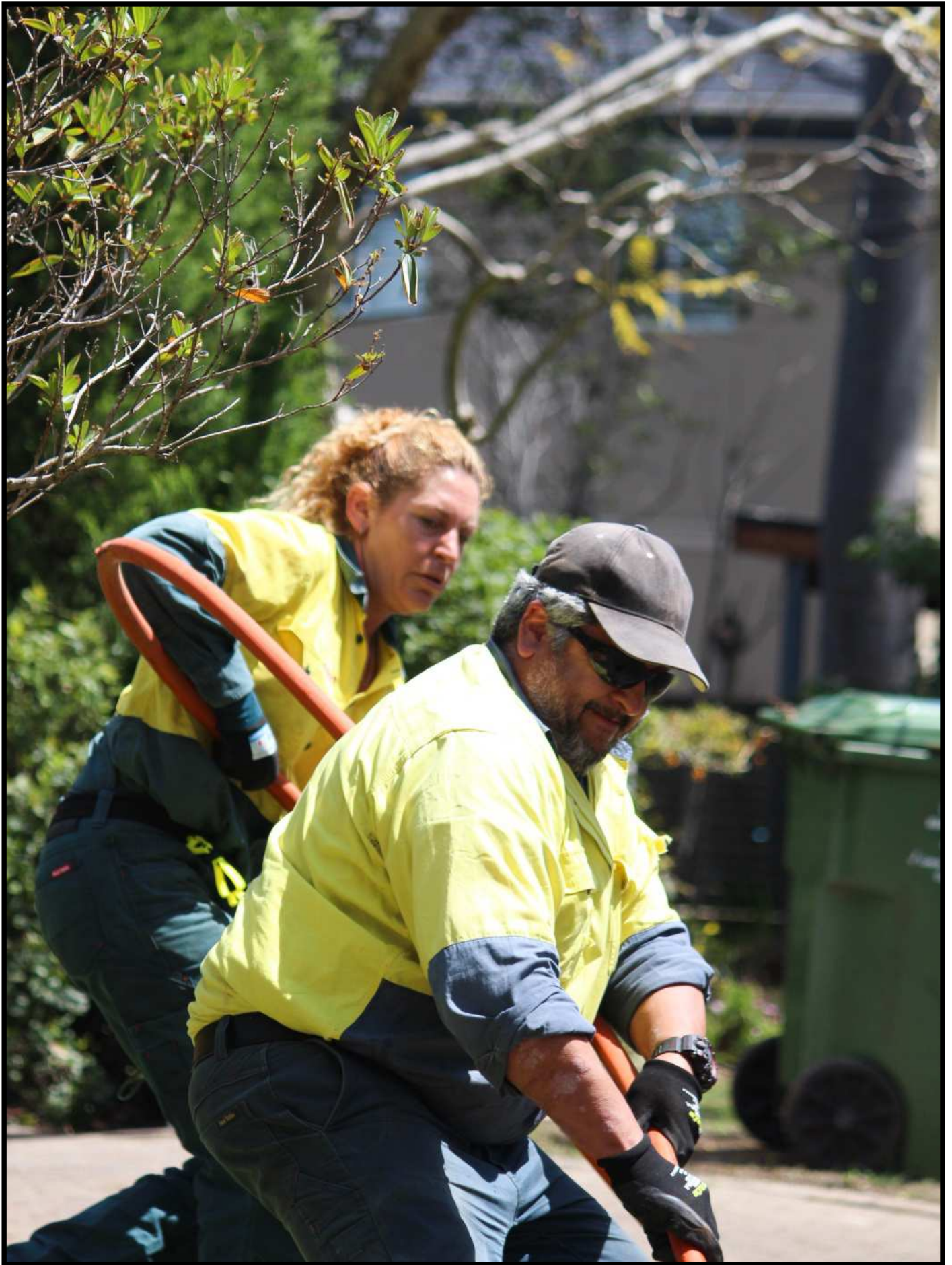
Ku-ring-gai Council operations staff completing drainage works.
