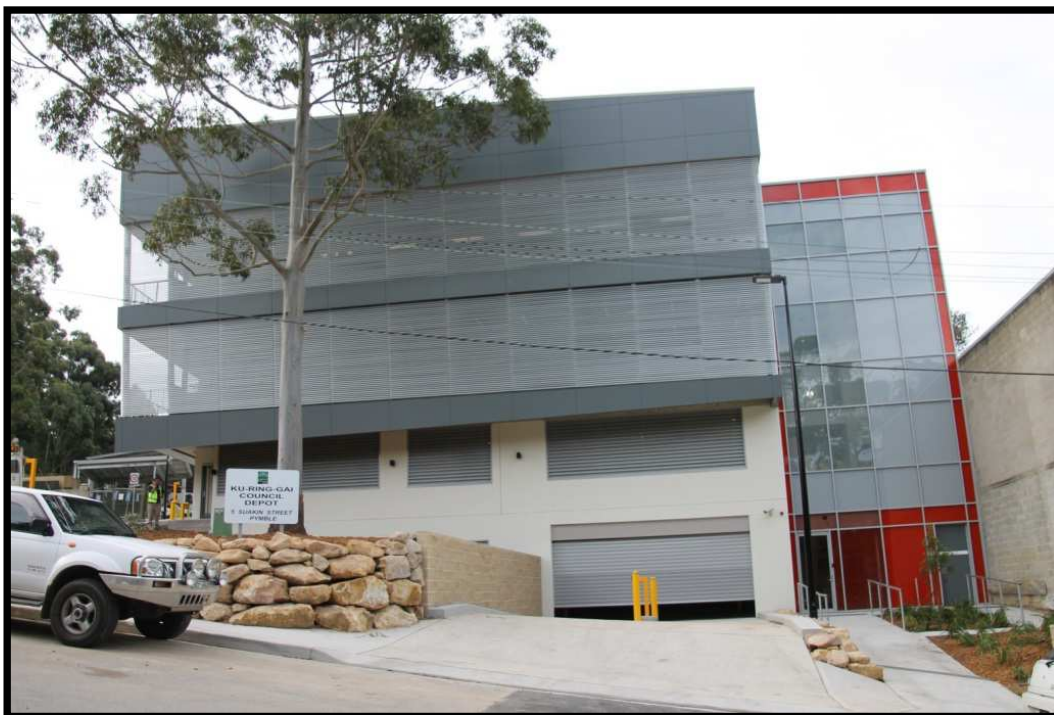
Ku-ring-gai Council Depot, Suakin Street, Pymble.
