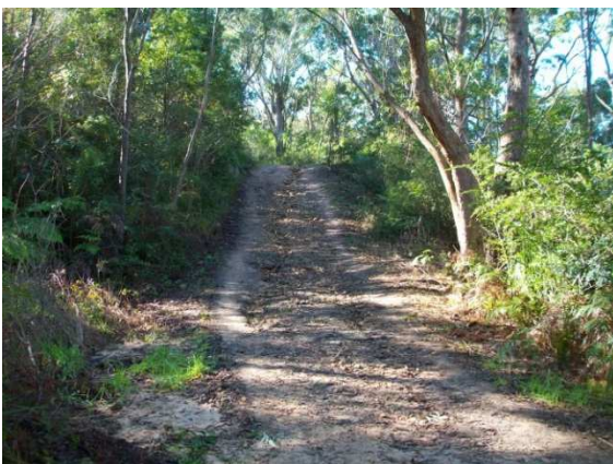
Fire trail upgrade – before
