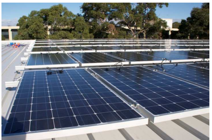
Solar panel installation
