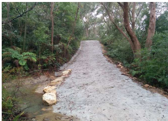
Fire trail upgrade – after
