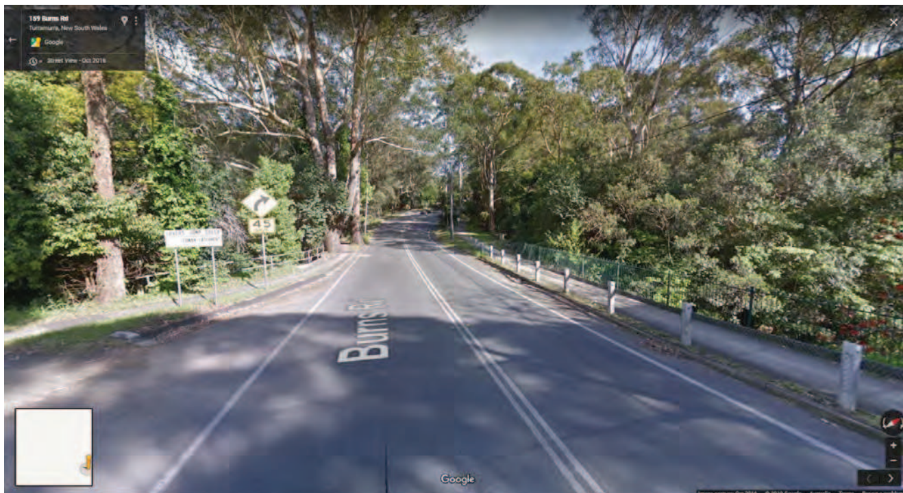
Figure 9-36 Existing defacto traffic barrier on downstream side (right-side of photo) of Burns Road crossing of Lovers Jump Creek (source: google StreetView). A 5m sheer drop to the right of green fencing, then a 10m waterfall drop.
