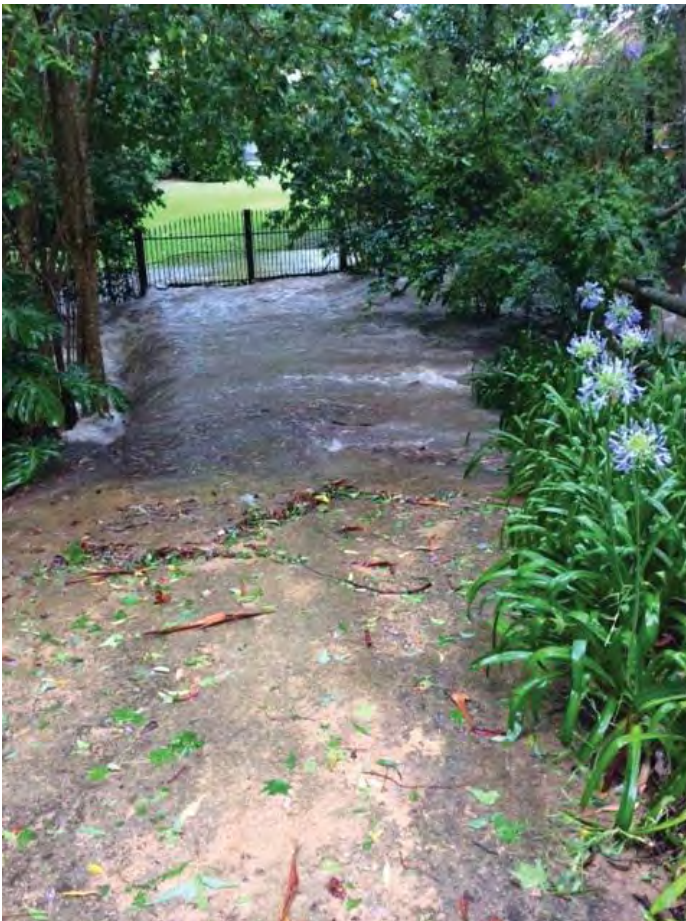
Plate 2-5. December 2014 event, showing overtopping of a driveway crossing with property cut-off from vehicular access.
