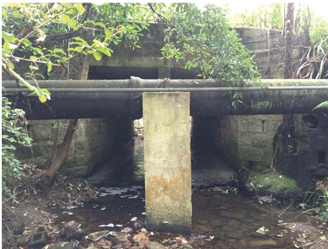
Plate 3-1 Water mains pipe partially obstructing The Chase Road culverts
