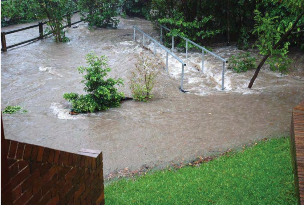
Plate 2-5. December 2014 event, showing overtopping of a driveway crossing with property cut-off from vehicular access.
