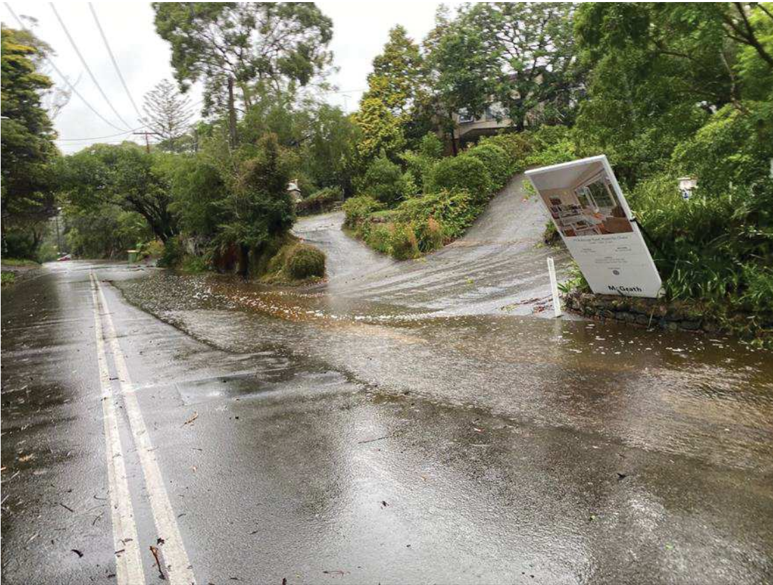
Figure D.2 Ponding on street in Roseville Chase during February 2020 storm (photo courtesy A.Adamovich)
