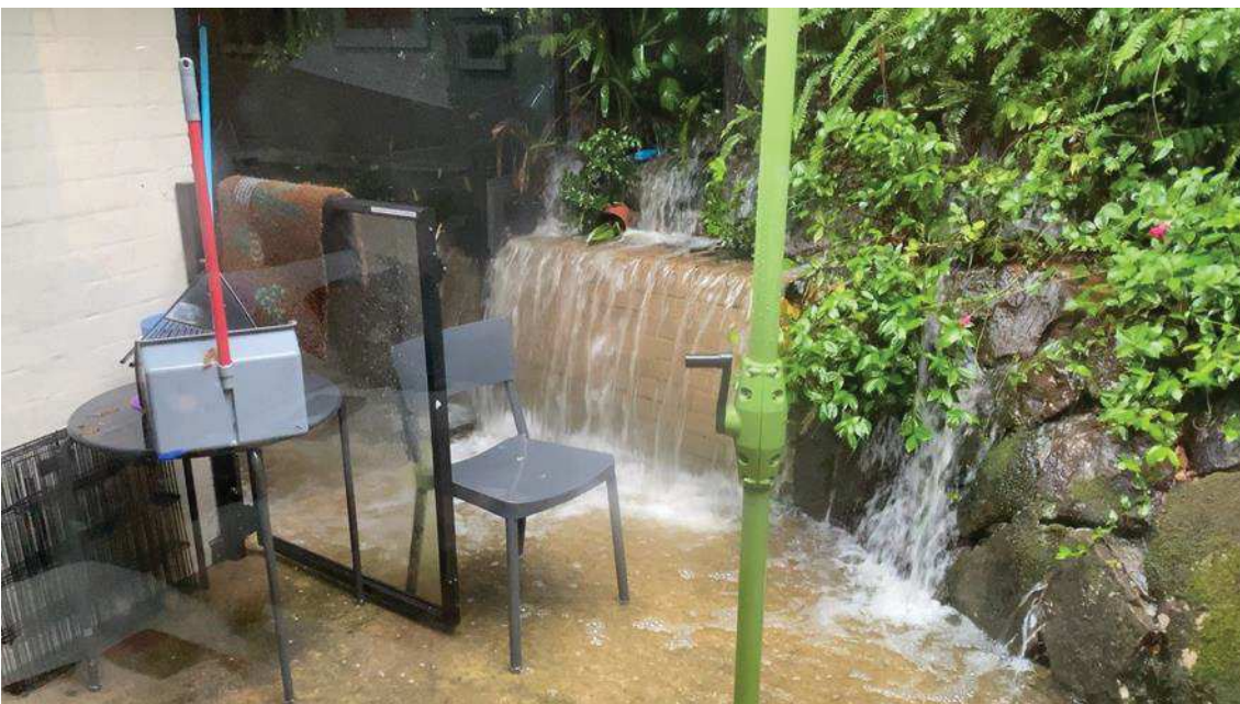
Figure D.3 Runoff into property in Roseville Chase during February 2020 storm (photo courtesy A.Adamovich)
