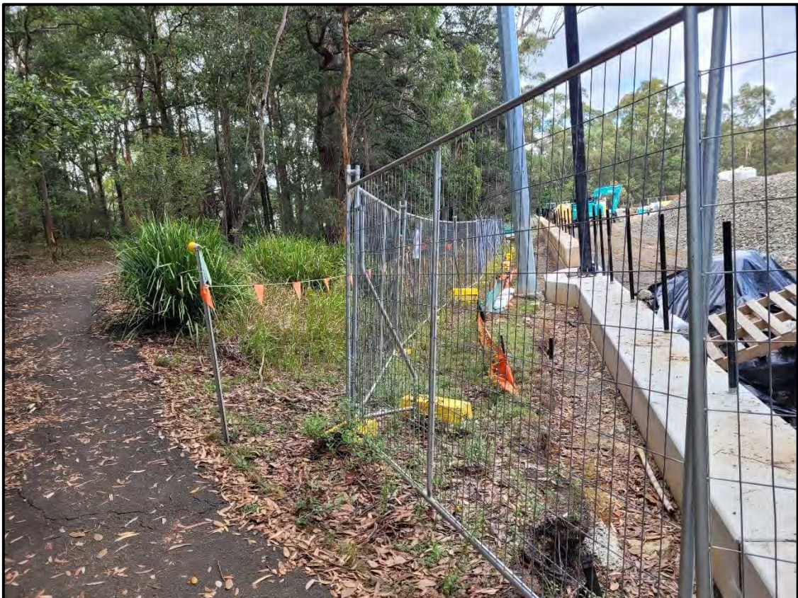
Figure 1-3 Southern edge of the Subject Site facing south, south-west showing the location where the existing footpath would be rejoined with the proposed footpath.
