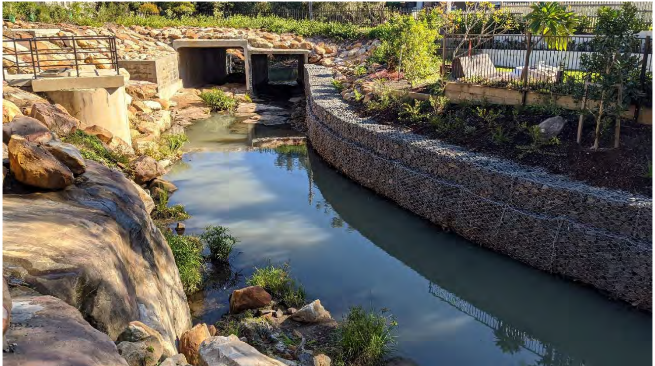
Figure 5-3 Gabion baskets installed along Dairy Creek
