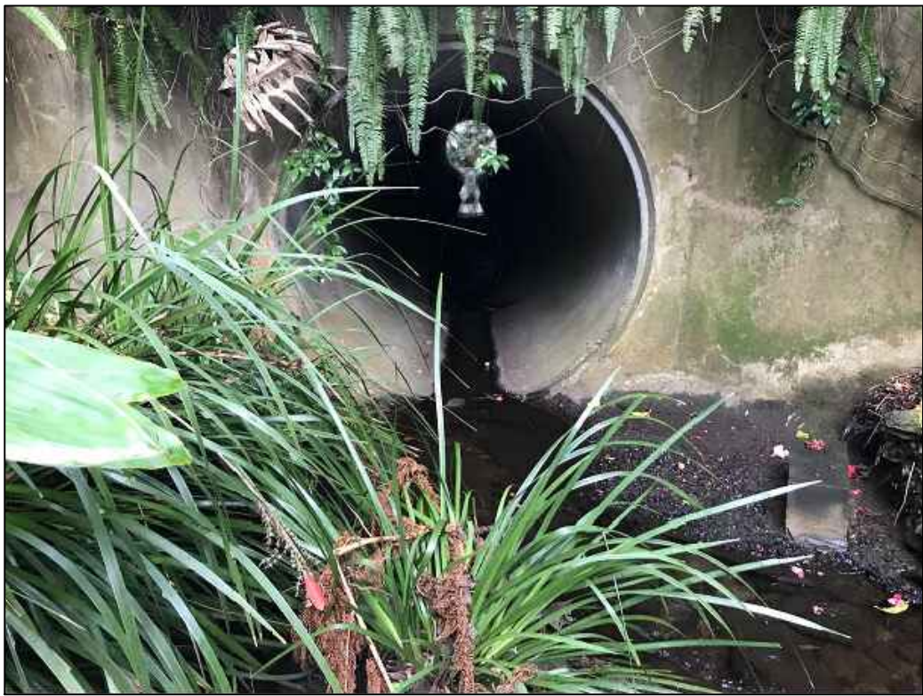
PHOTO F2 CULVERT - DOWNSTREAM
