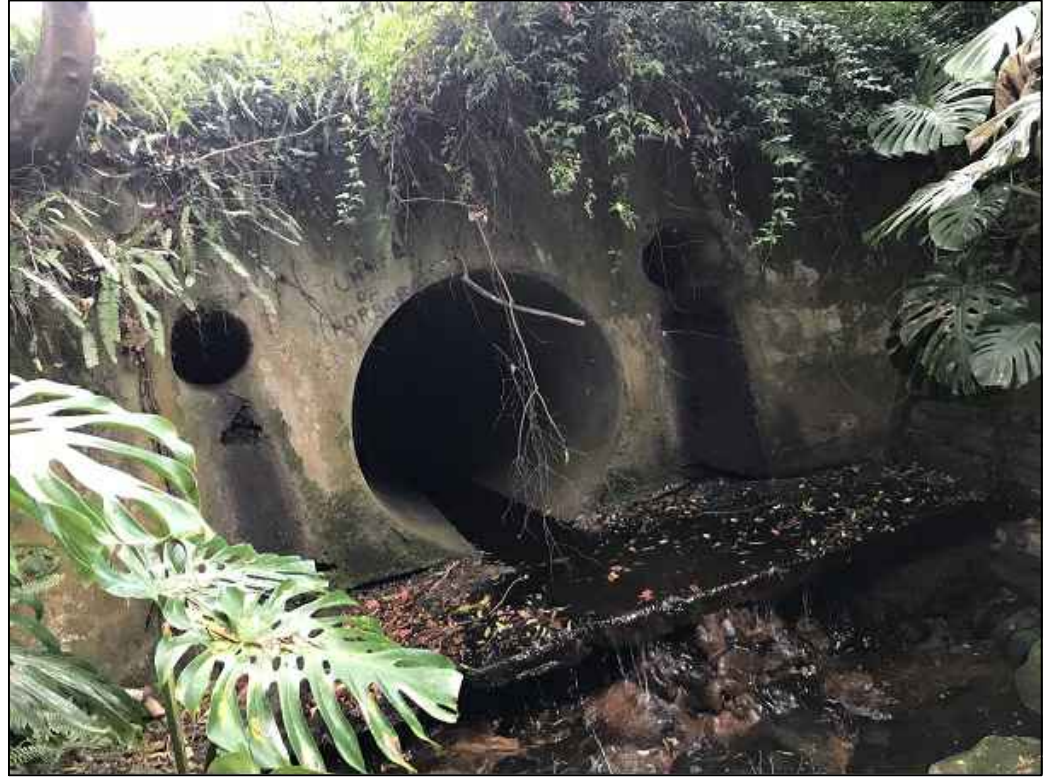
PHOTO G1 CULVERT WATERWAY
