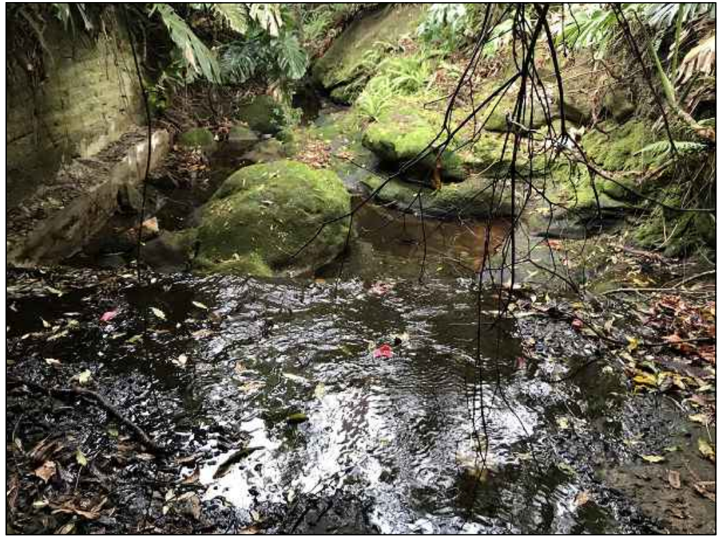
PHOTO G1 CULVERT - DOWNSTREAM
