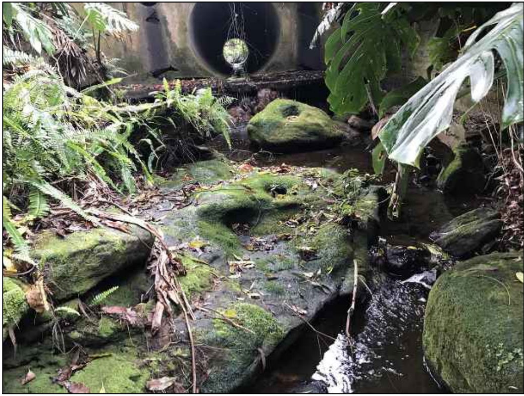
PHOTO G1 - UPSTREAM
