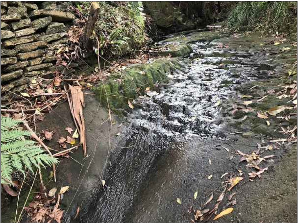
PHOTO A2 CULVERT - UPSTREAM
