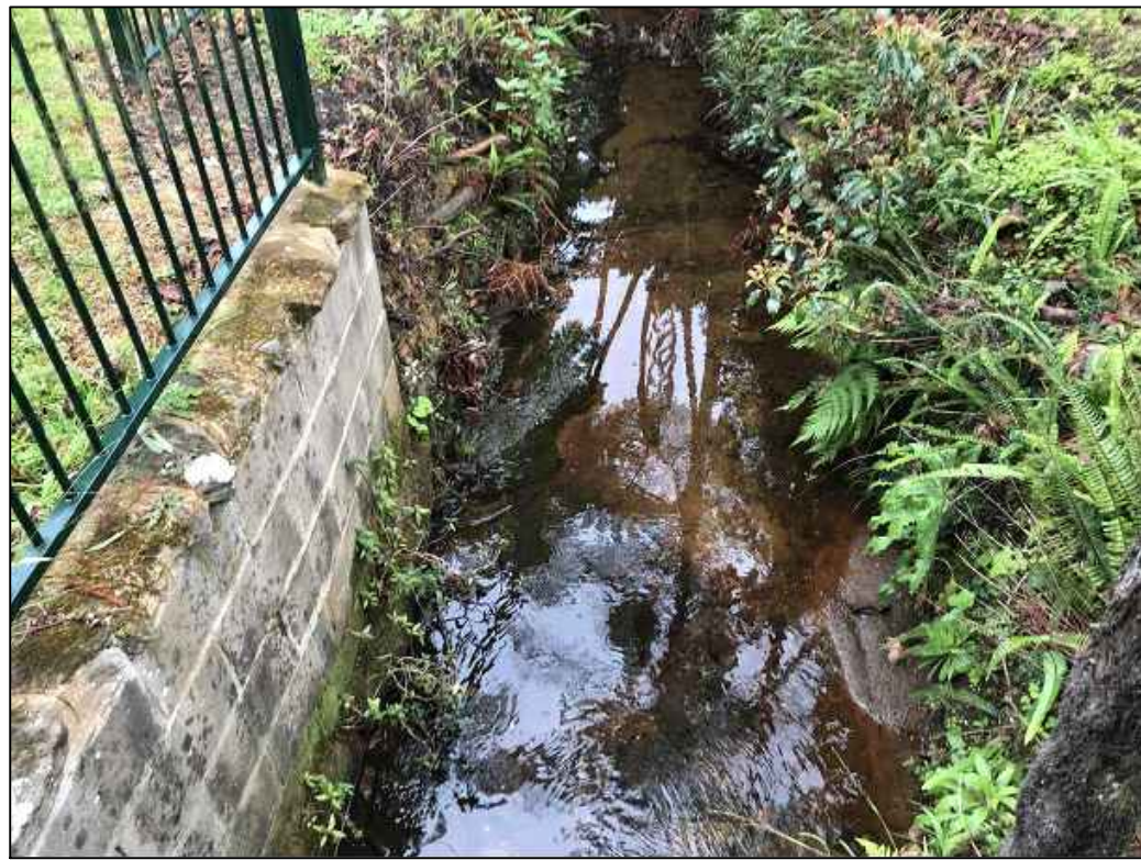
PHOTO BETWEEN F1 & F3 - DOWNSTREAM
