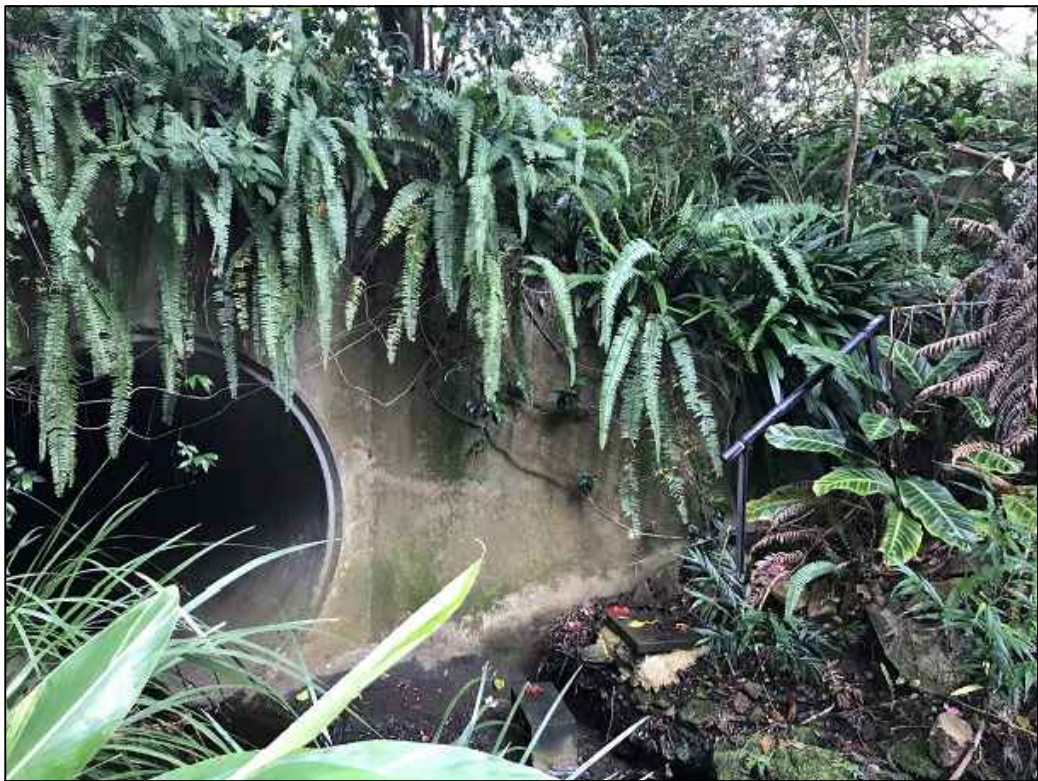
PHOTO F2 CULVERT - DOWNSTREAM
