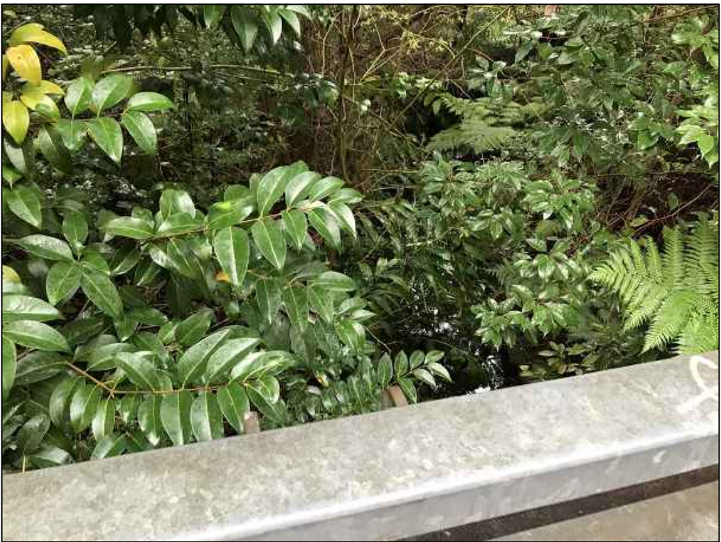
PHOTO D2 TROON PLACE BRIDGE - TOP - DOWNSTREAM
