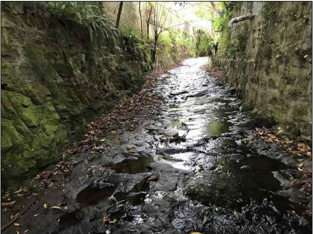
PHOTO G8 CULVERT - UPSTREAM
