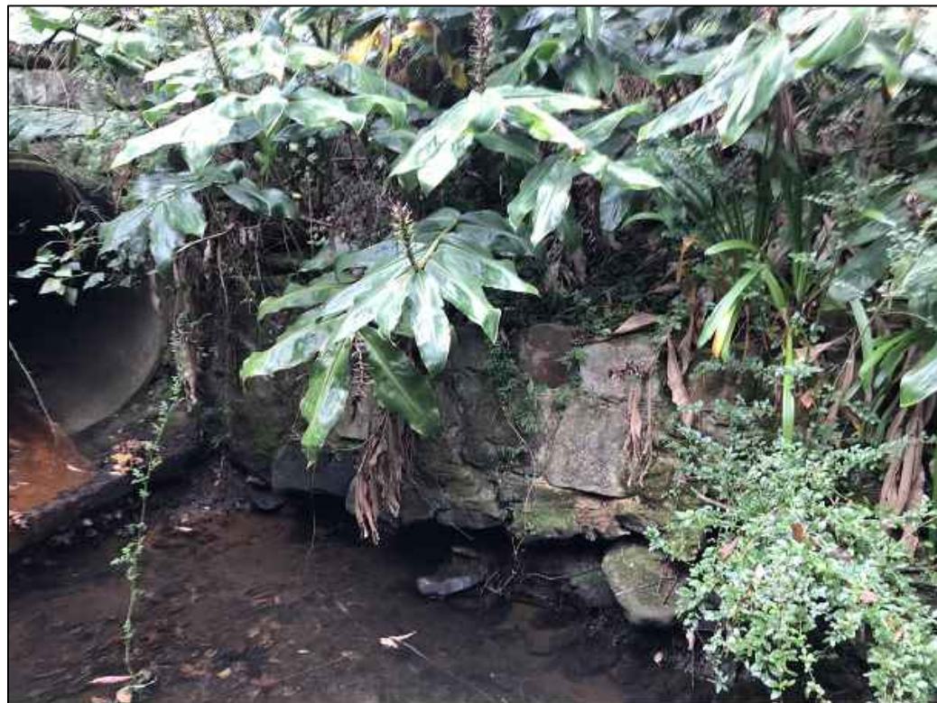
PHOTO A1 CULVERT - WATERWAY
