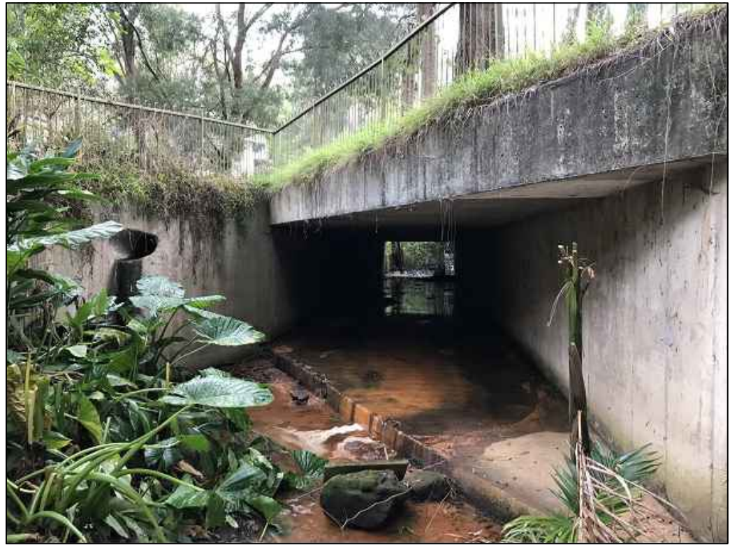
PHOTO D1 CULVERT - UPSTREAM
