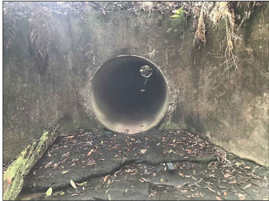
PHOTO B1 CULVERT - UPSTREAM
