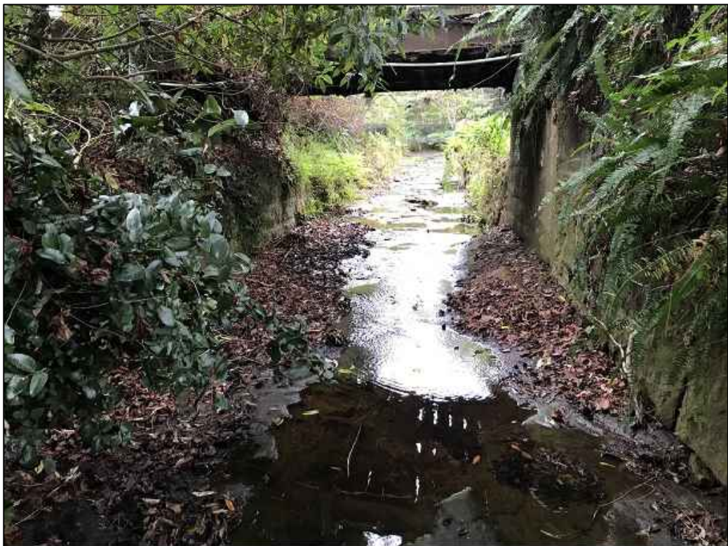
PHOTO G7 - UPSTREAM
