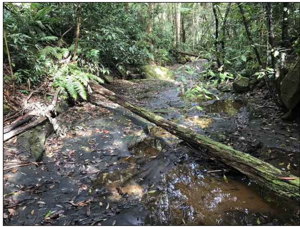
PHOTO B1 CULVERT - DOWNSTREAM
