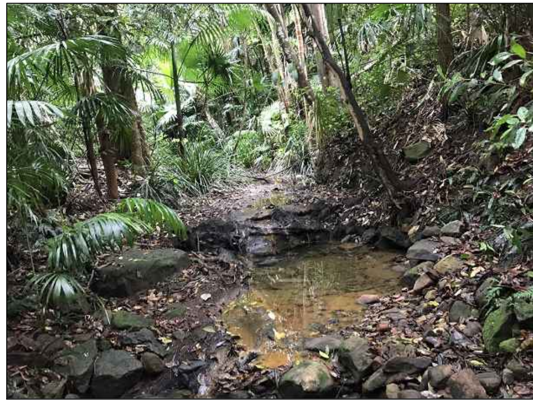
PHOTO B2 CULVERT - UPSTREAM
