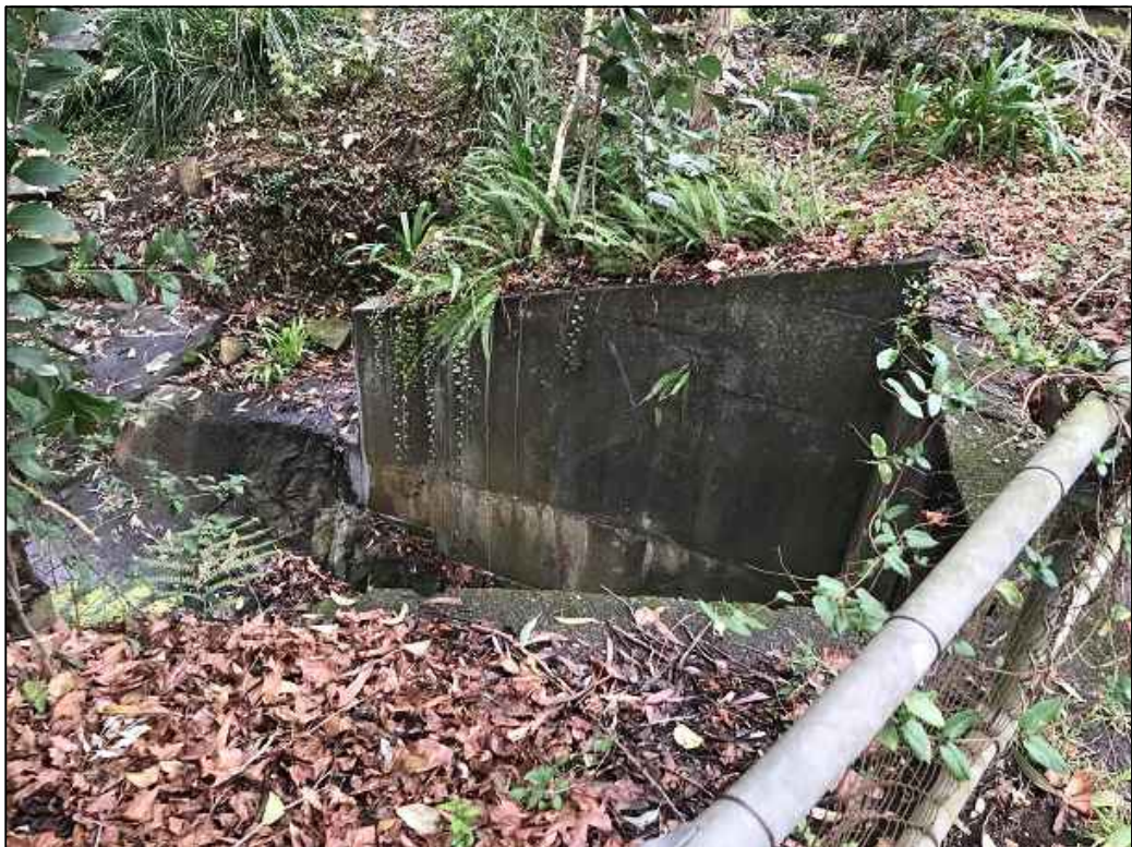
PHOTO A2 CULVERT - TOP
