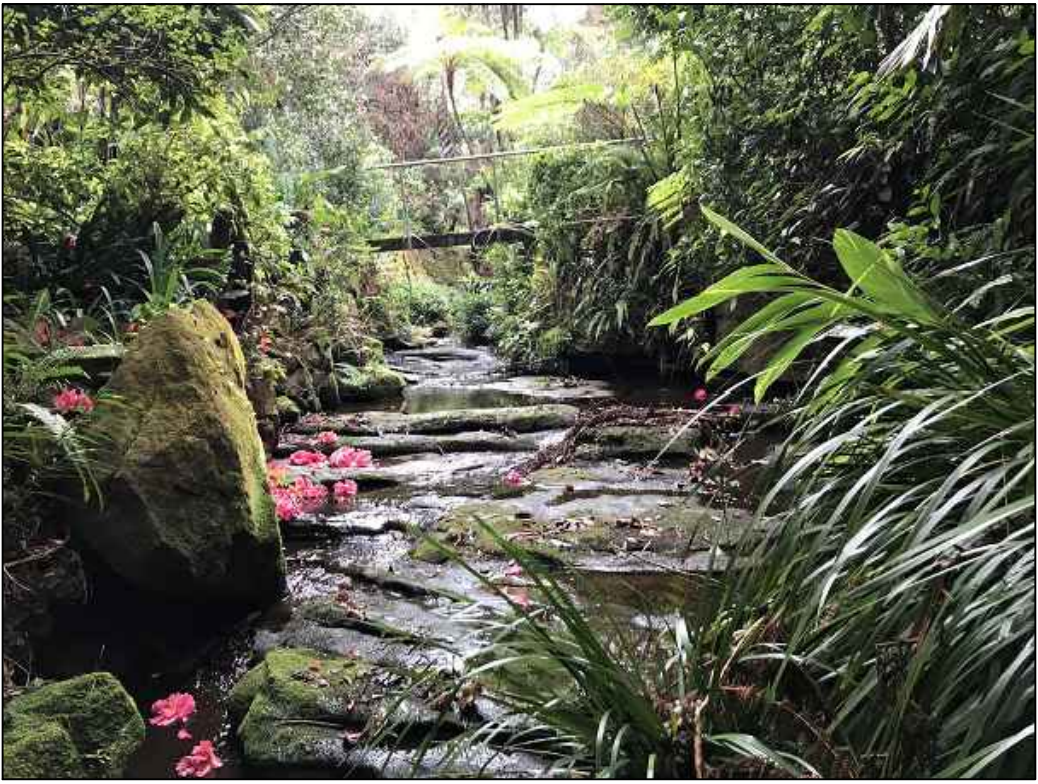
PHOTO F2 CULVERT - UPSTREAM
