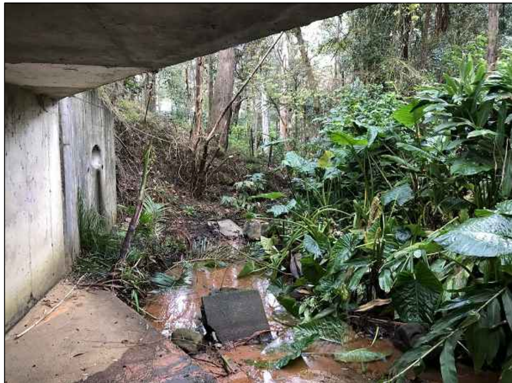
PHOTO D1 CULVERT - DOWNSTREAM
