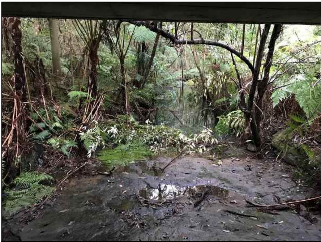
PHOTO D2 TROON PLACE BRIDGE - UPSTREAM
