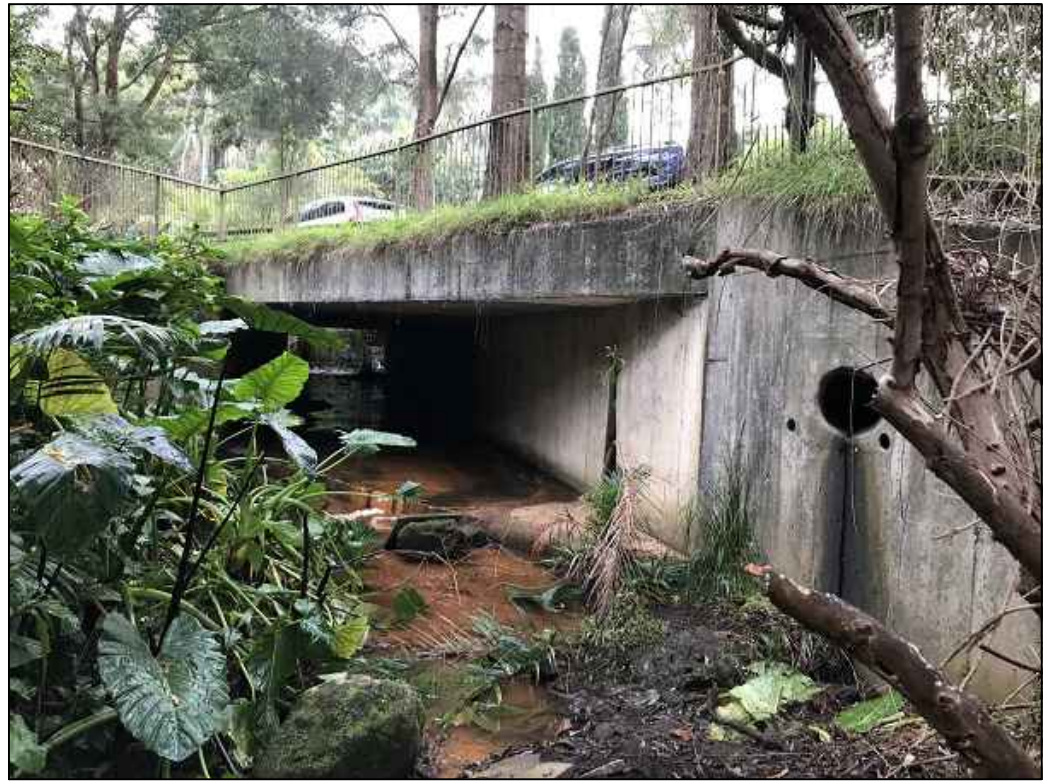
PHOTO D1 CULVERT HEADWALL - UPSTREAM
