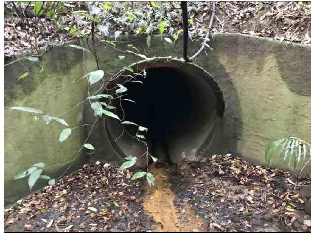
PHOTO B2 CULVERT - DOWNSTREAM
