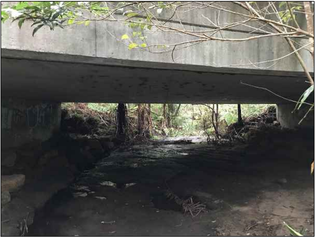
PHOTO D2 TROON PLACE BRIDGE - UPSTREAM
