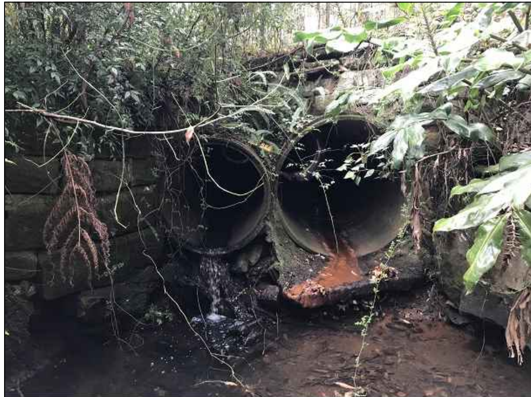
PHOTO A1 CULVERT - UPSTREAM
