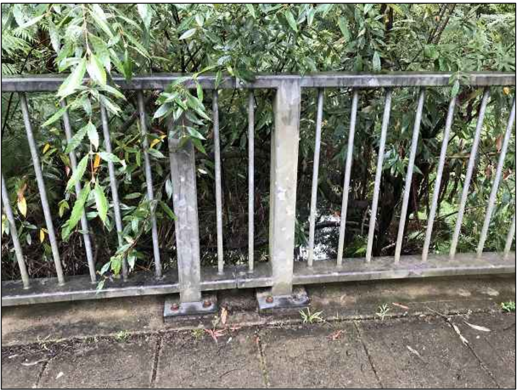
PHOTO D2 TROON PLACE BRIDGE - TOP - UPSTREAM
