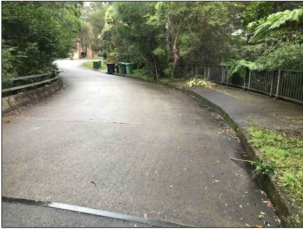
PHOTO D2 TROON PLACE BRIDGE - TOP
