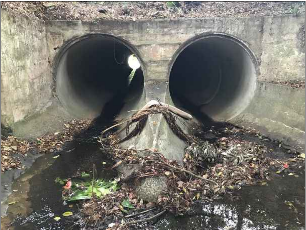
PHOTO G8 CULVERT - DOWNSTREAM
