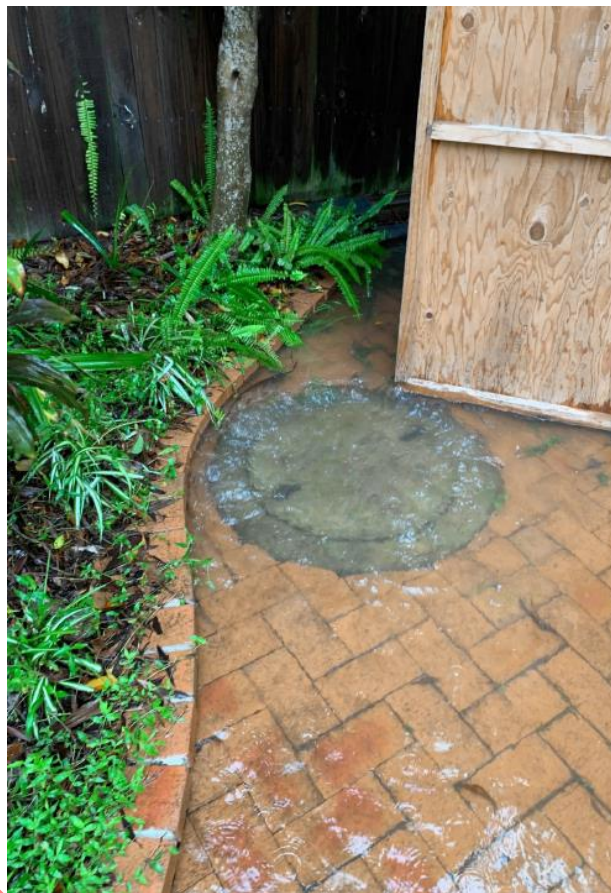
Photo 11: 9 February 2020 flooding in the back yard of a property on Yarrara Road, West Pymble, caused primarily by sewer overflows (ID 061)
