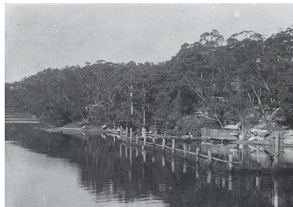
Photo 3. First Roseville Baths 1924. Note simple enclosure of timber posts & netting, natural shoreline & men's dressing shed at south-eastern end of pool. (Ku-ring-gai Library Photo 1335: Cazneaux Collection)
