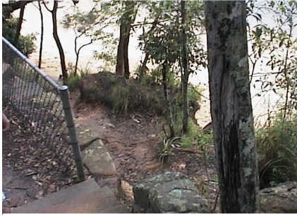
Photo 1. Eroded short-cut track.
