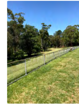
F Chain mesh fence
