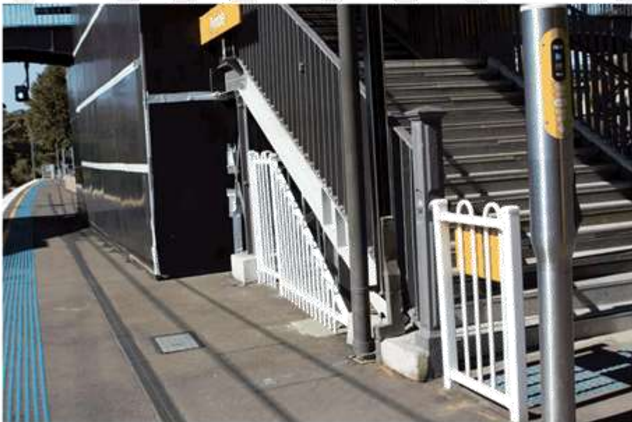
Plate 4.21 Footbridge stairs to platform with example of Newel post (RPS 2020)
