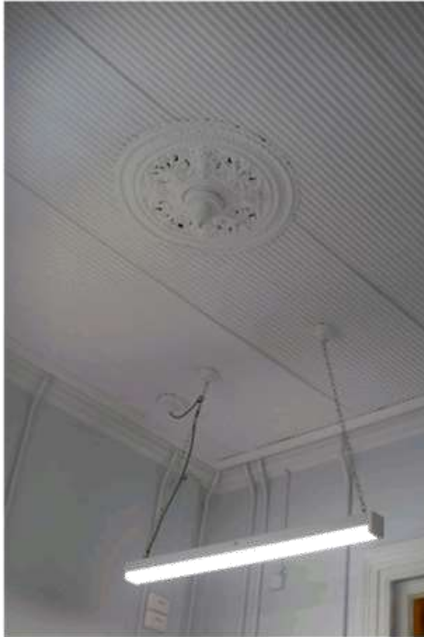
Plate 4.11 Ceiling of Ticket Office showing ceiling rose, plaster cornice and lighting (RPS 2020)
