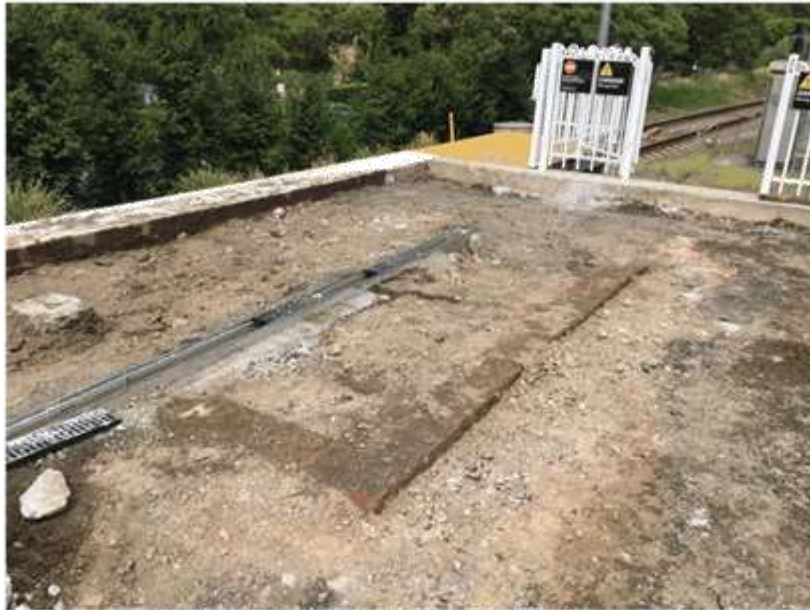
Plate 5.2 Brick footing exposed at the eastern end of the platform, looking northeast (Extent 2018:5)
