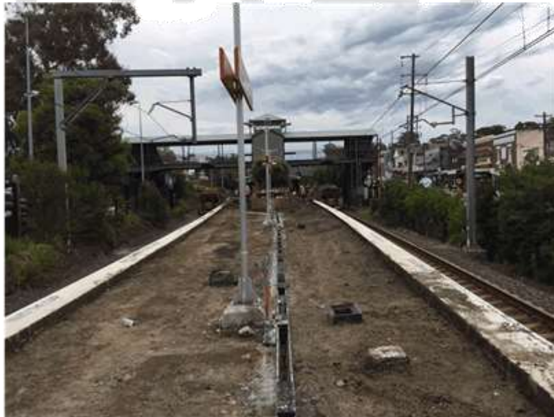
Plate 5.1 Platform resurfacing 2018 (Extent 2018:5)
